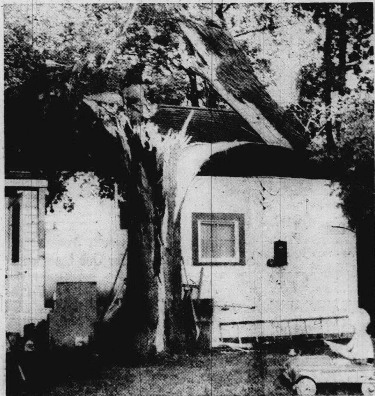
LAST THURSDAY'S short but violent windstorm felled a giant elm that crushed the roof of a home at 9821 Beck Rd. It belonged to Nick Zander of Nick's Barber Shop. The tree split and fell in all directions. Damage inside the home was surprisingly
