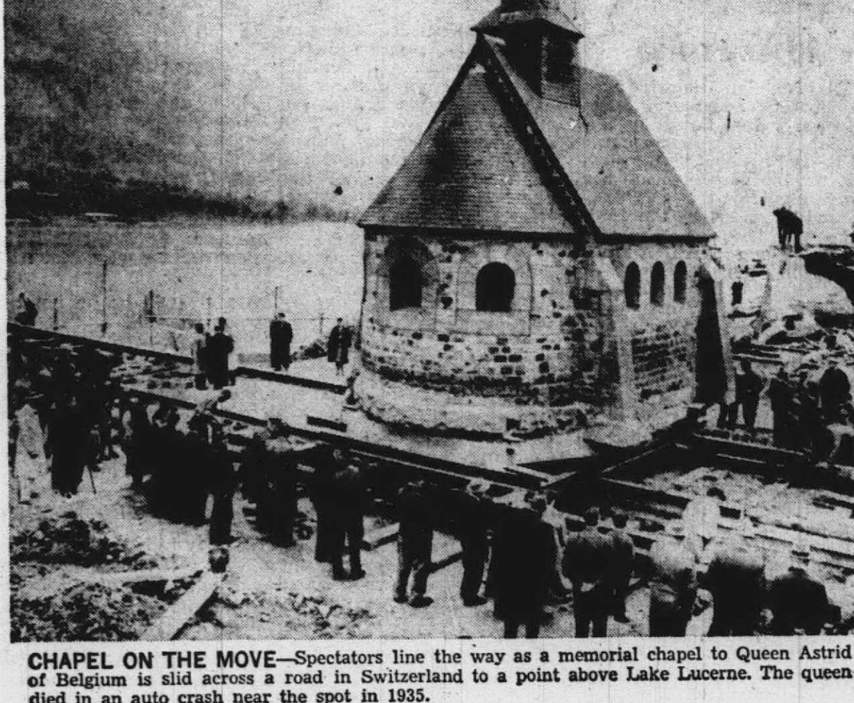
CHAPEL ON THE MOVE—Spectators line the way as a memorial chapel to Queen Astrid of Belgium is slid across a road in Switzerland to a point above Lake Lucerne. The queen died in an auto crash near the spot in 1935.
