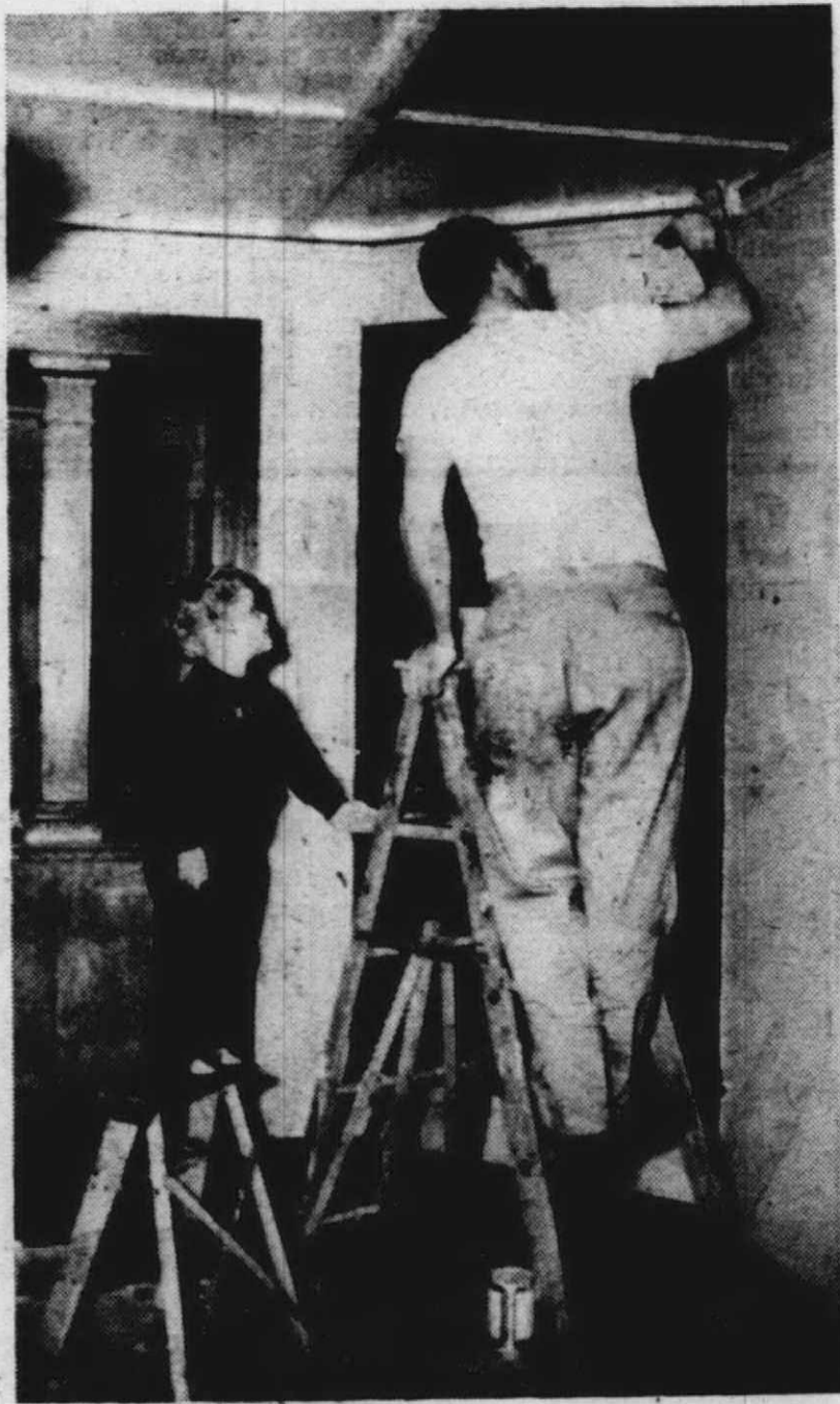
PLENTY OF HELP — A brush is the utensil for painting woodwork (photo above) and a roller makes short work of the walls. Although the paint brush will never be completely displaced, the roller method of painting, as easy as it is, has prompted many a novice to repaint his home's interior.
