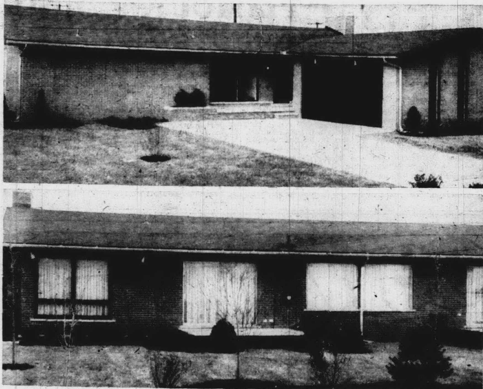
THE 1960 IDEA HOME is a study in contrasts as well as a complete departure from the conception of making the front seem more attractive than the rear. The front view (at the top) shows the garage in front of the L-shaped brick veneer structure, with only the three panels of amber glass in the entrance hall and the other three in the side of the garage breaking up the somewhat somber appearance. In the rear, however, the home is almost all clear glass, as the bottom photo indicates. From left to right are the large double windows in the living room, the eight-foot doorwall off the dining area, the large double windows in the children's room and the six-foot doorwall off the master bedroom. There are two patios, one off the dining area and the other off the master bedroom. The home, located at Farmington and Six Mile Roads, Livonia, will be open to the public for only eight weeks, January 9 through March 6. Visitors will have an opportunity to win the home by estimating the number of nails contained in a replica.
