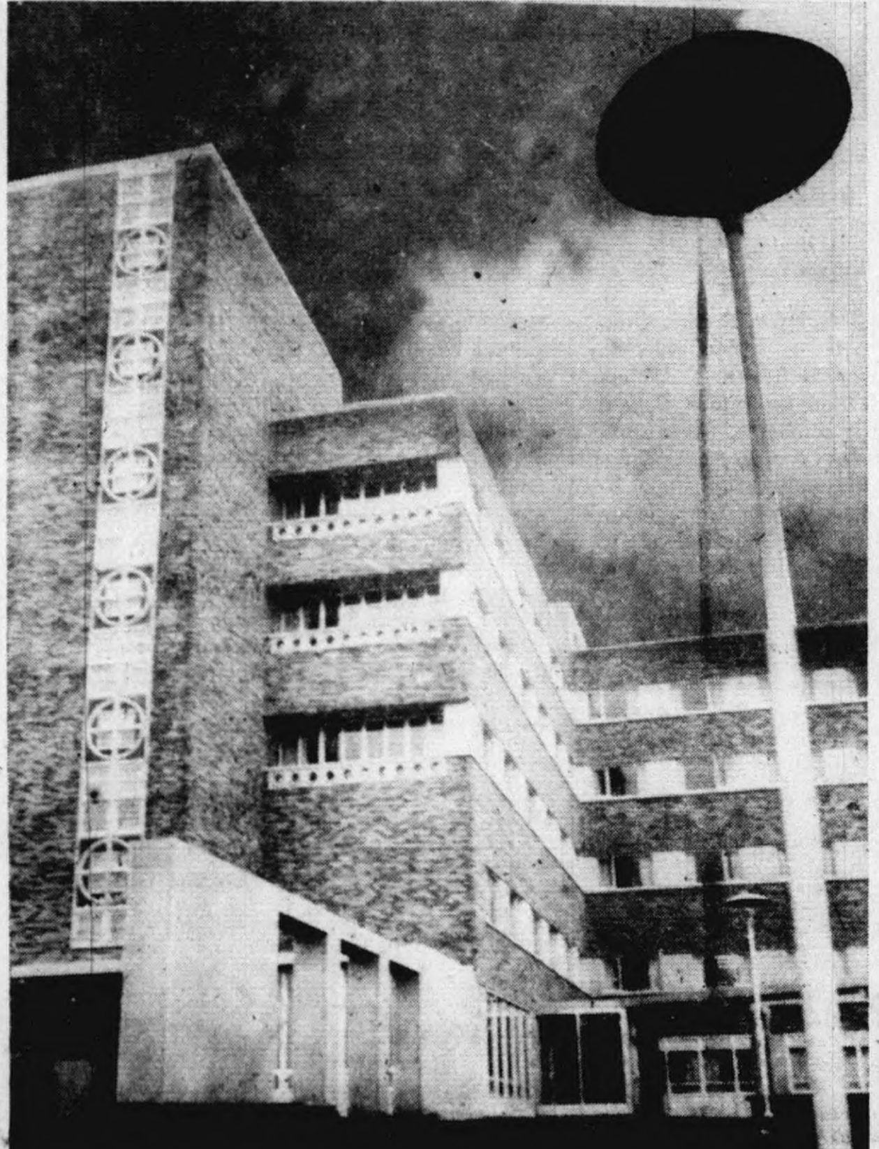
TOWERING FIVE STORIES above the flat land of western Livonia is St. Mary Hospital, the area's first major hospital. Throngs of local people were
