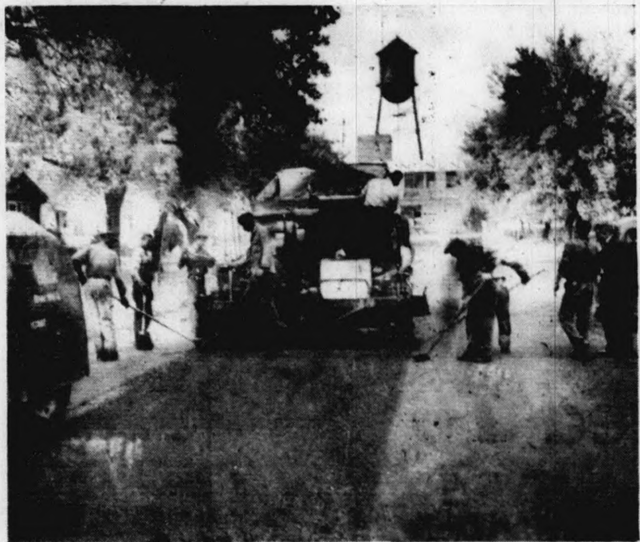
PAVING OF three streets, including the much-used Harvey St. from Ann Arbor Trail to Junction, is being completed this week. The asphalt paving machine is shown moving on Harvey toward
