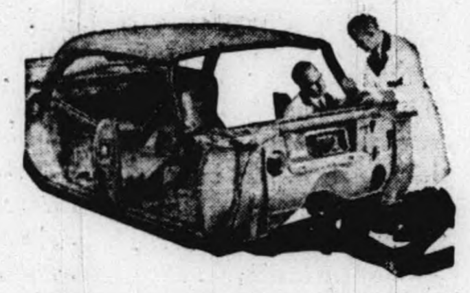
Unibody Construction: frame flows into the body, makes it twist as strong, twice as quiet—surrounds you with silent strength.
