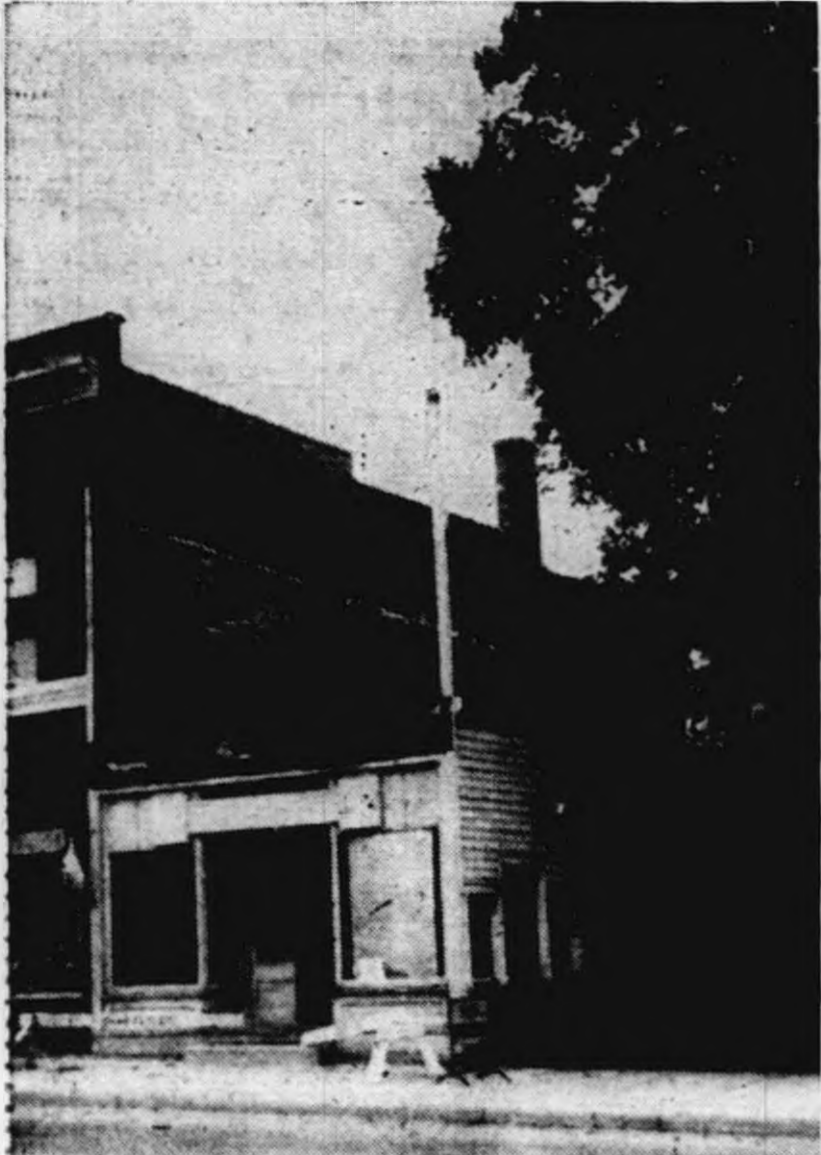
THIS OLD BUILDING between Schraders Funeral Home and Fisher's Shoes has been razed. Schraders will build a second chapel and improve its office space on the lot. The second chapel will make it possible to hold two funerals nearer together, owner Edwin Schrader announced. The job will be completed in 120 days. Architecture will blend with the present funeral home.
