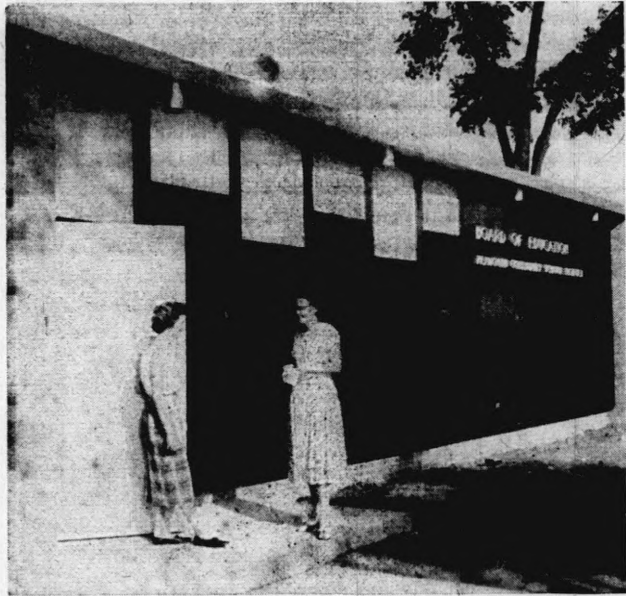
ALTHOUGH some finishing touches are still being made, the school district's new administrative offices are now in use on S. Mill St. beside the Junior High. Here, Mrs. Barbara Christensen
