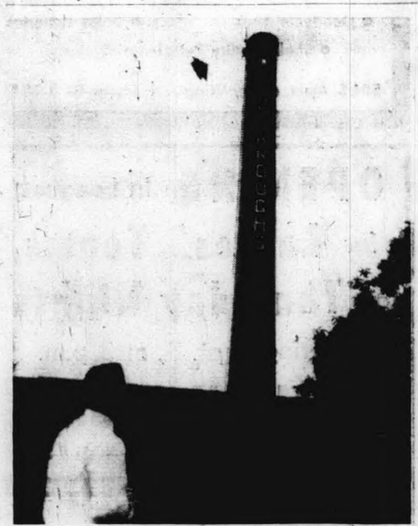
THAT SPECK AT the top of the smokestack at Burroughs Plymouth Division is a daring young man from the Custodias Construction Company Inc., of Royal Oak, who is busy replacing the concrete cap that is designed to protect the top of the chimney from the weather. At the same time workers installed new lightning rods. The operation was completed last week.
