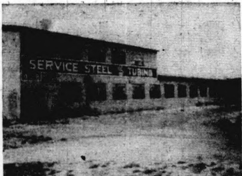
THIS WAS CONSIDERED the most up-to-date type of factory when it was constructed in 1914 to make motor cars. Located on Farmer St., it now has broken windows and decaying timber.
