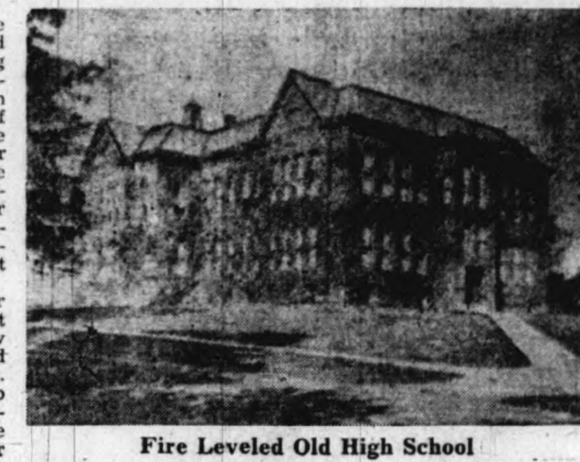
Fire Levelled Old High School
