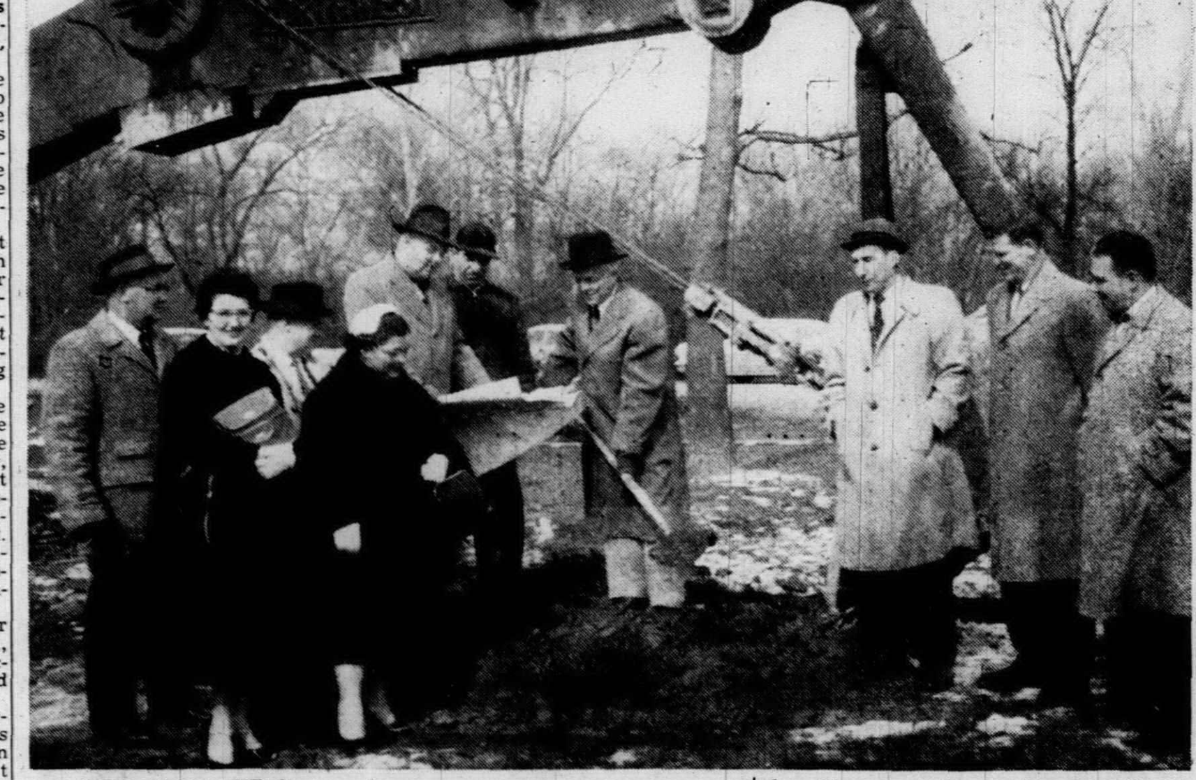
START OF THE first major sewer construction in Plymouth Township's history called for a groundbreaking ceremony Wednesday morning. Supervisor Roy Lindsay is shown turning over the first shovelful of ground where the sewer empties into the Middle Rouge Interceptor at the western edge of Newburg Lake. The project will cost $578,900 and will take about seven months. From left are Trustee Louis Norman, Clerk Rosalind Broome, Trustee C. V. Sparks, Treasurer Elizabeth Holmes, Engineer Herald Hamill, contractor Tony D'Angela, Supervisor Lindsay, Warren Worth, engineer of highways for the Road Commission; J. Winghart, Road Commission engineer; and Wayne Rice of the Road Commission legal division.
