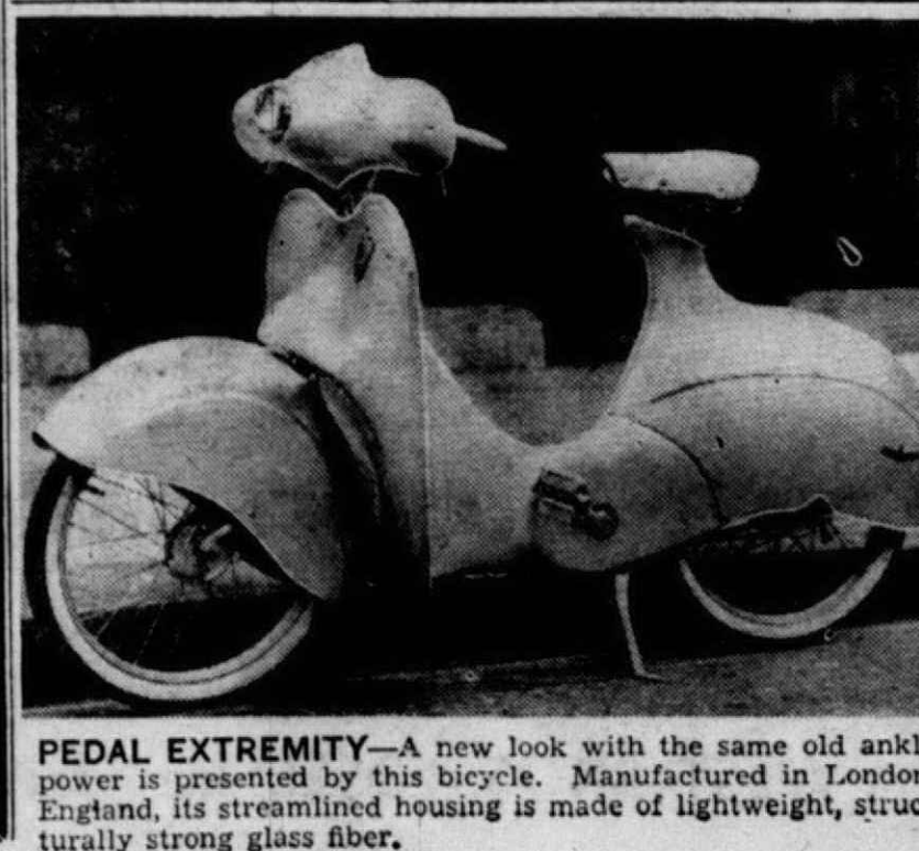
PEDAL EXTREMITY—A new look with the same old ankle power is presented by this bicycle. Manufactured in London, England, its streamlined housing is made of lightweight, structurally strong glass fiber.
