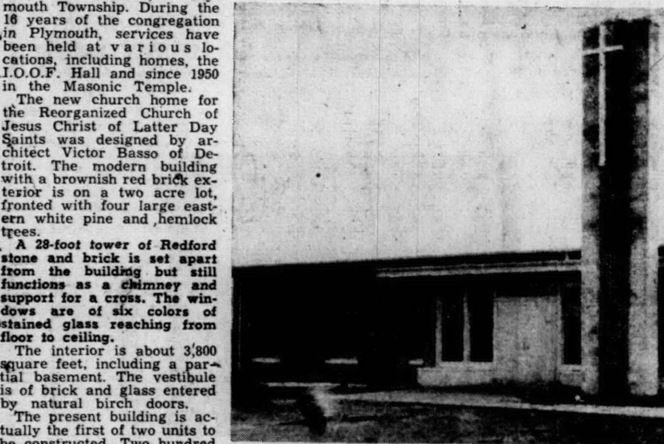
DEDICATION OF this church by the Reorganized Church of Jesus Christ of Latter Day Saints will take place this Sunday afternoon. The new edifice is on Schoolcraft Rd. The free-standing tower is also a chimney.
