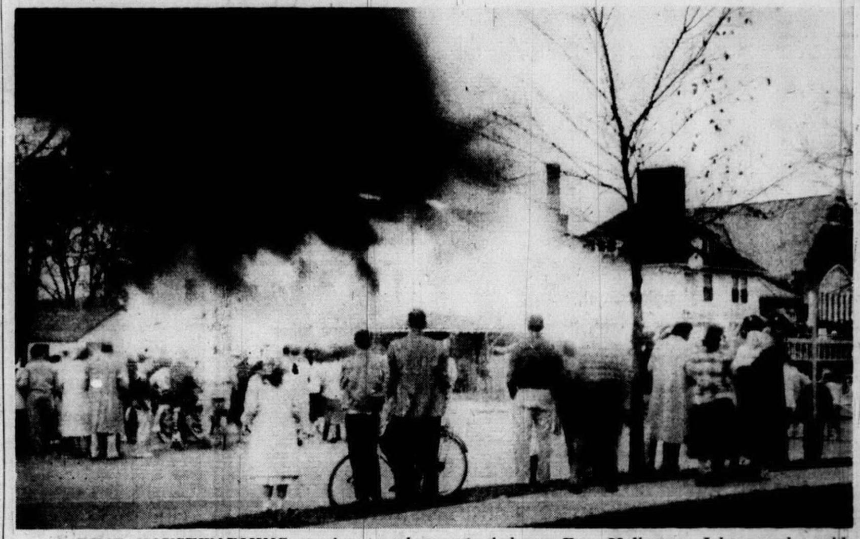
A REAL HOUSEWARMING session took place last week when firemen deliberately burned down an old home at Church and Adams streets. Owned by First Methodist Church, the house was leveled to make way for possible future expansion. With the church parsonage only 25 feet away, most spectators expressed hope that firemen knew what they were doing. Least
