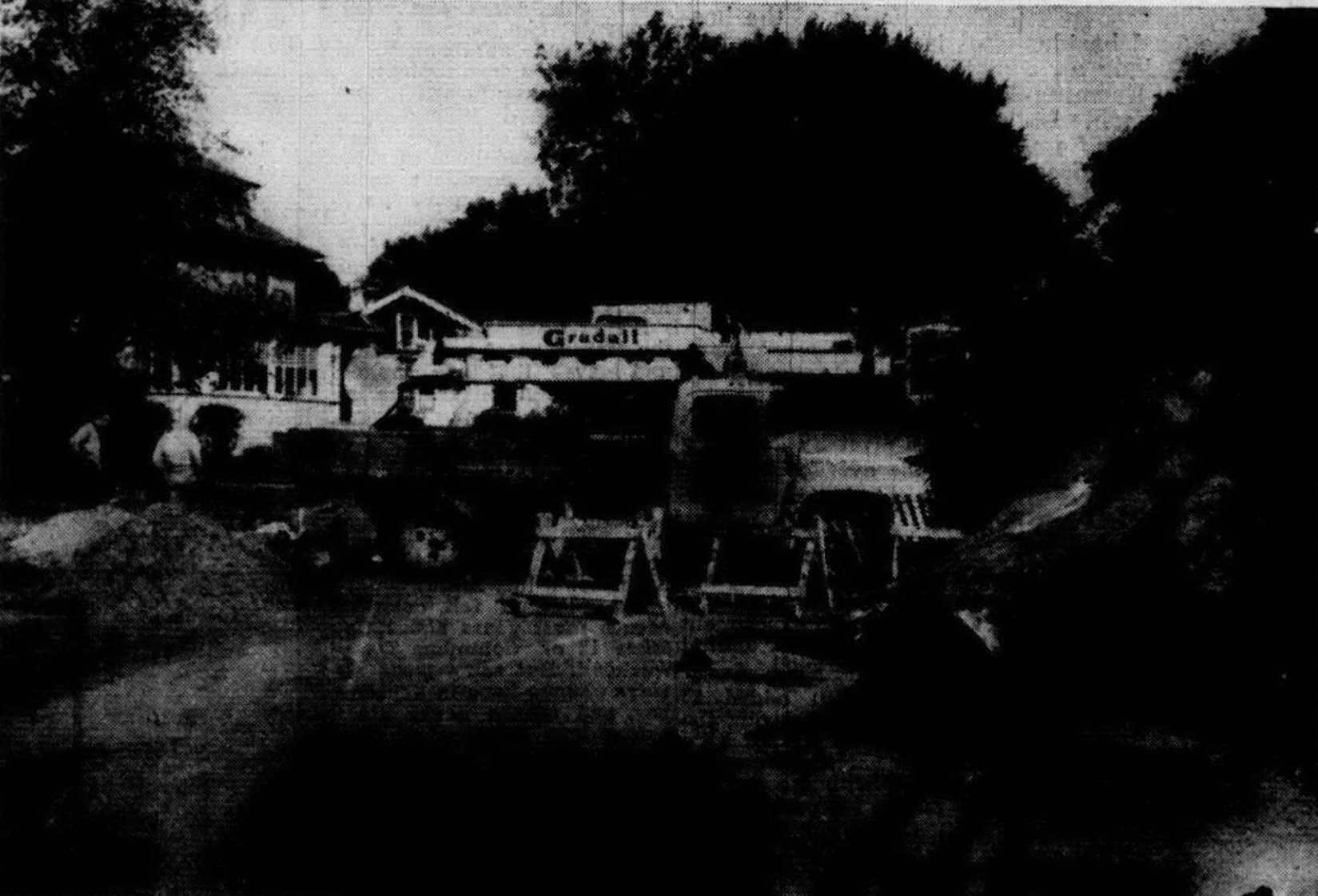
WORK ON the South Main St. widening and paving project is moving forward with trees now removed. Sewers must be adjusted, the pavement ripped up and a new foundation laid be-
