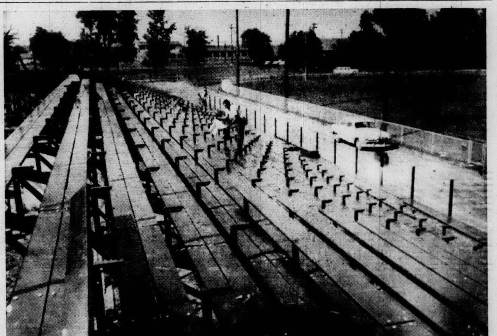
NEW BLEACHERS are now ready for the kick-off of the 1958 Plymouth High football season on Friday, Sept. 19. The bleachers were completed this week on the west side of the field. Holding 1,416 people, the stands cost $12,127.
