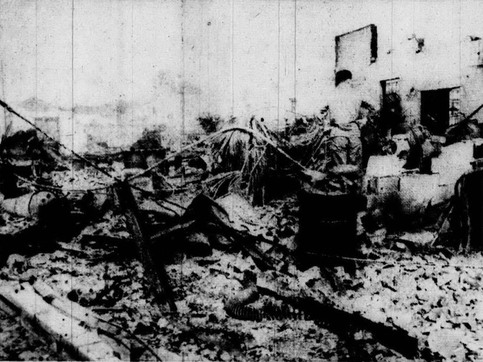
YESTERDAY HE was working, today he is jobless because of a fire that destroyed the Peerless-Industries Co. plant on North Territorial Rd. This employe was one of 40 working for the plumbing specialty plant. He is shown surveying the still smoking ruins Wednesday morning.
