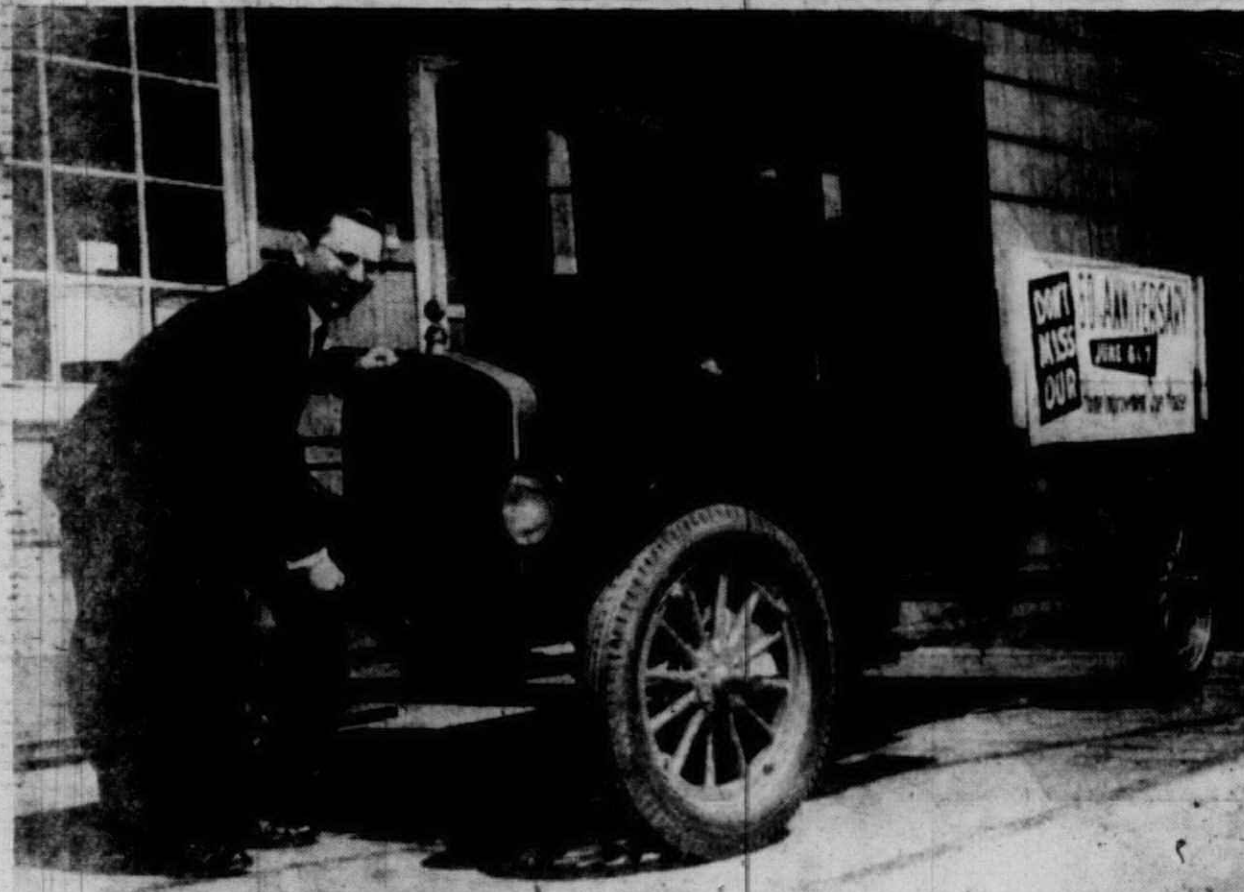
HAULING LUMBER in horse-drawn wagons and later in trucks such as this 1927 Model T are all part of the eras that Plymouth Lumber & Coal Co. went through.
