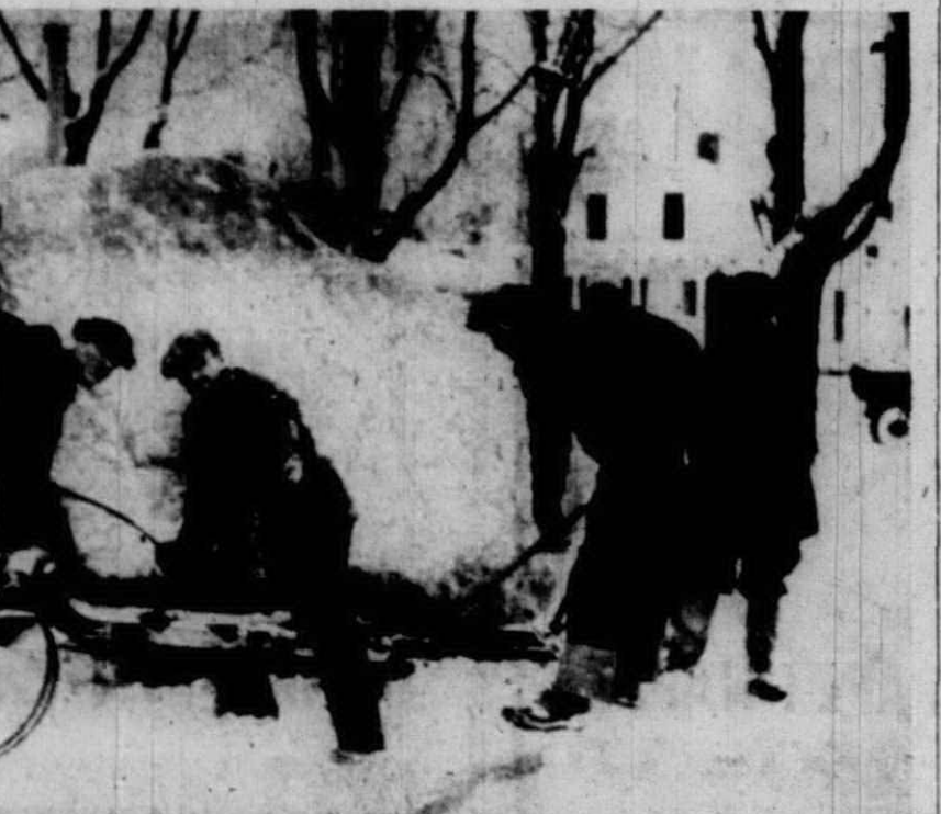
ON A SNOWY morning in February 1935 the giant boulder used for Plymouth Rock was moved into place. It was found while excavating for the railroad overpass on Northville Road and was moved by the Ex-Servicemen's Club. This photograph taken by Wood Studio looks toward Penniman Ave. where the Penn Theatre now stands.
