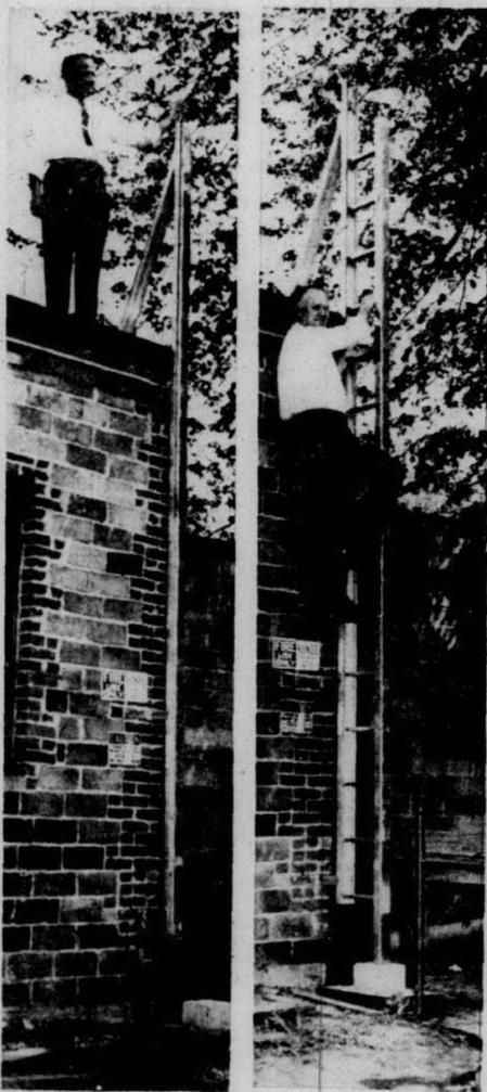
**INVENTOR** Dan Spence demonstrates his first fire ladder installation at Saxton's Farm Supply. Standing on the roof, he pulls a handle (left) on top of an object that looks something like a down-spout. In an instant a ladder springs forth and the inventor climbs down. The ladder has been given city approval. Offices are located on the second floor of the building's front half.
