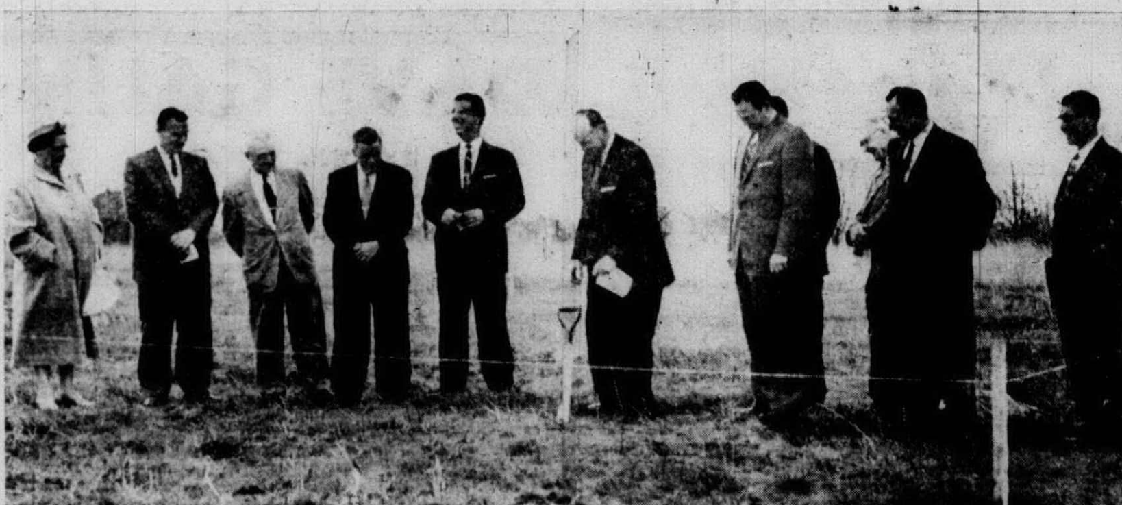
SOD WAS TURNED Sunday, April 20 on the site of the new Reorganized Church of Jesus Christ of Latter Day Saints at the Schoolcraft-Bradner intersection. Present at the groundbreaking serv-
