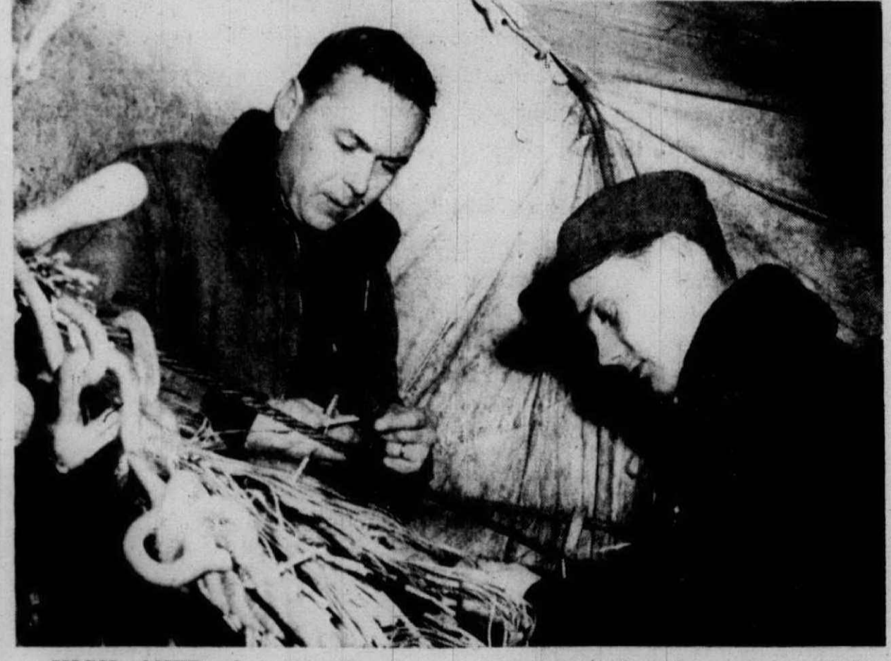
HIGH OVER the city streets, Dale Hirth and Fred Briggs work in a Michigan Bell splicers' tent interconnecting the tiny wires which carry calls to and from the dial exchange.
