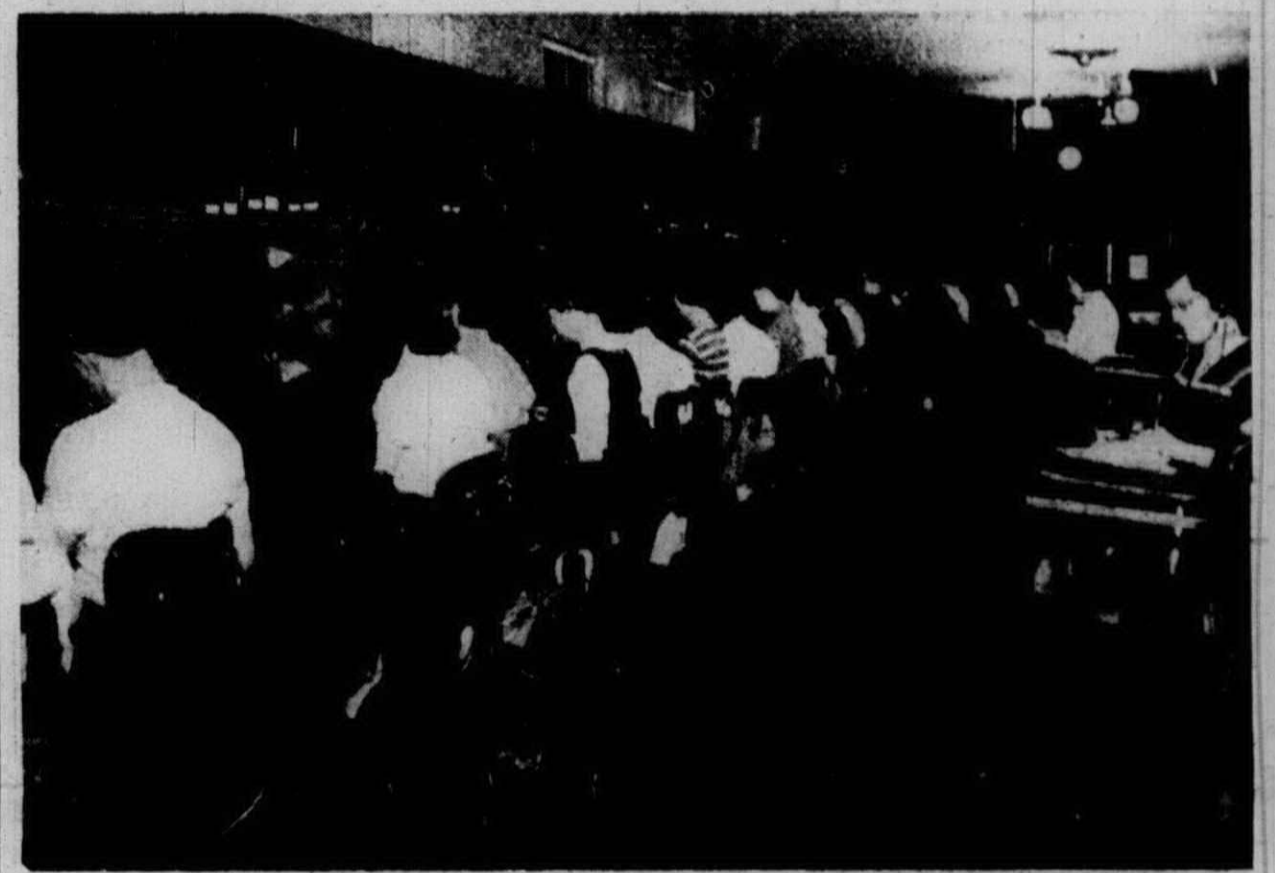
SOON TO BECOME a part of communications history in Plymouth is this manually operated switchboard located in the Ann Arbor Trail equipment building. The board has served Plymouth many
