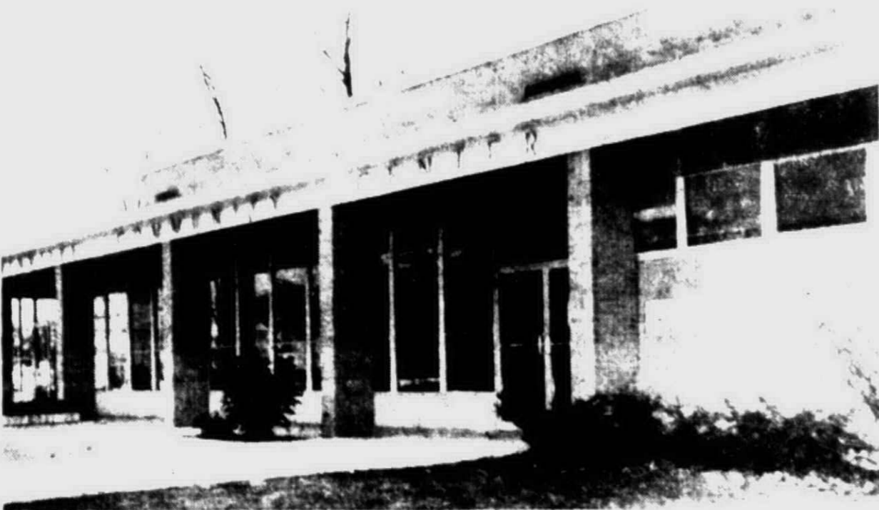
NORTHVILLE'S Community Center is an attractive, modern building near the center of town. But unlike Birmingham's Community building, it has rather limited "community" use. It is operated by the board of education and is used mainly for school functions.
