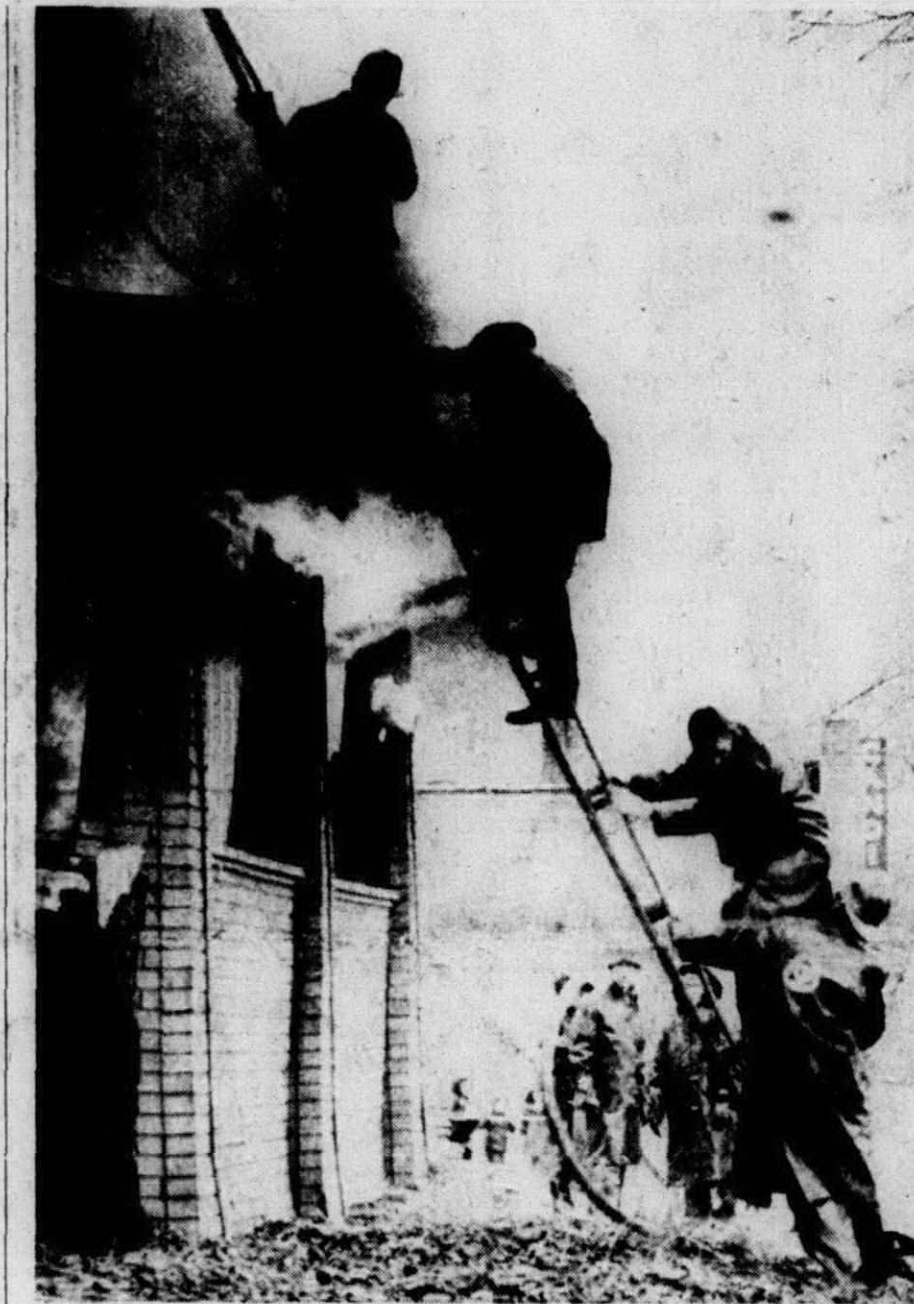
HOT-FOOTING it down a ladder as flames shoot around them were three firemen caught atop porch roof as the underside burned in last week's firefighting demonstration. The three were watching for outbreaks of fire upstairs while the firefighting demonstration was going on downstairs. Suddenly flames shot around edges of the porch roof and the firemen hastily retreated, unhurt, to the ground.
