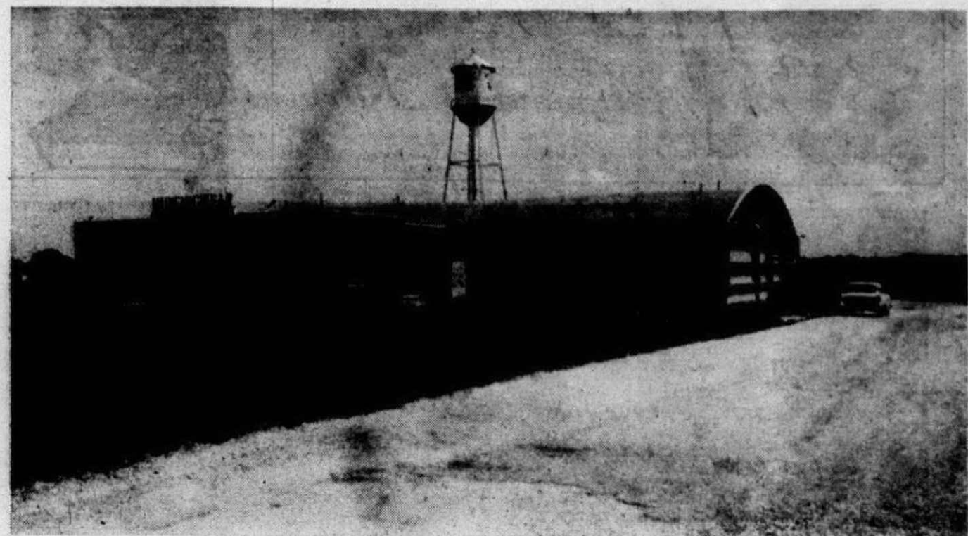
ONE OF THE new plants of Rogers, Arkansas is the Munsingwear plant. makers of nylon hosiery. A development plant will build the plant for Daisy.
