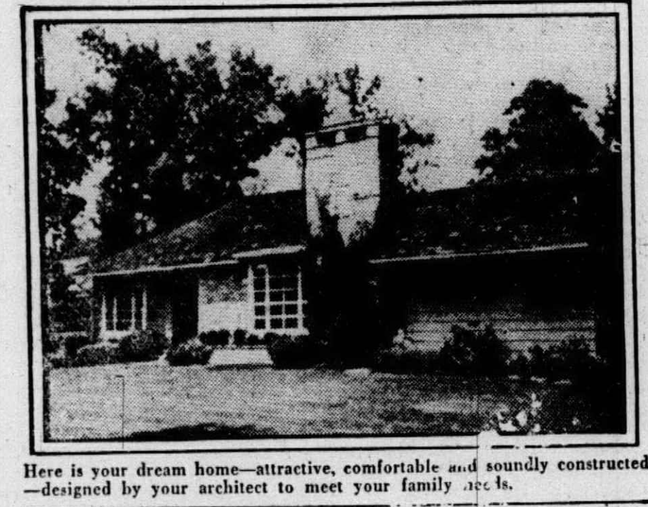
Here is your dream home—attractive, comfortable and soundly constructed—designed by your architect to meet your family needs.
