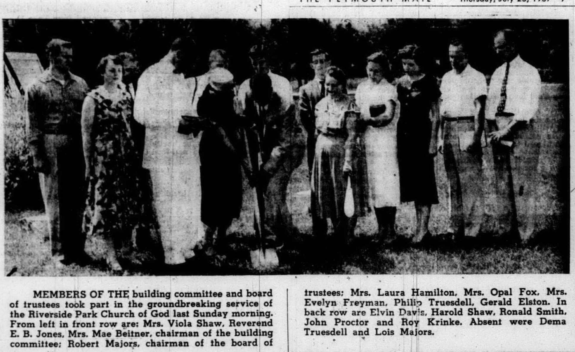
MEMBERS OF THE building committee and board of trustees took part in the groundbreaking service of the Riverside Park Church of God last Sunday morning. From left in front row are: Mrs. Viola Shaw, Reverend E. B. Jones, Mrs. Mae Beitner, chairman of the building committee; Robert Majors, chairman of the board of
