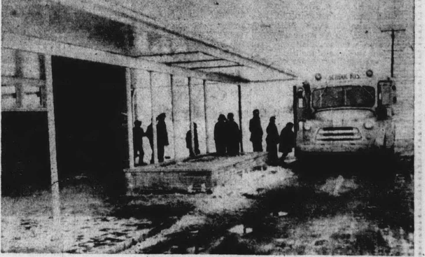
AMONG THE practical features of the new Gallimore Elementary schools is a bus loading port. Without standing in the rain or snow, youngsters can get on and off buses while under roof. Stone box in center of picture is for shrubs or flowers.
