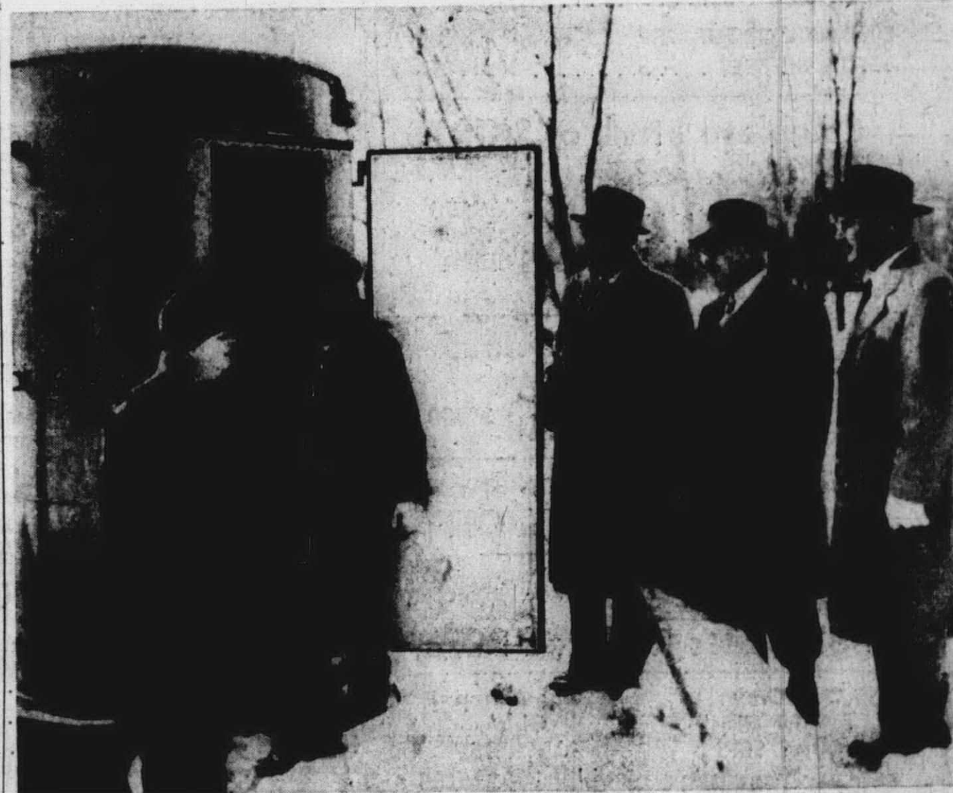
IT WAS too cold last week for any type of an official opening ceremony but some of those responsible for constructing the city's $600,000 sanitary sewer were pictured at the entrance to the pumping station. From left are Engineer Herald Hamill; Leon Holda, superintendent for the contractor; Mayor Russell Daans and City Manager Albert Glassford; and Jack Cooper of Plymouth, distributor for Smith-Lovelace corporation, sellers of the pumping unit.
