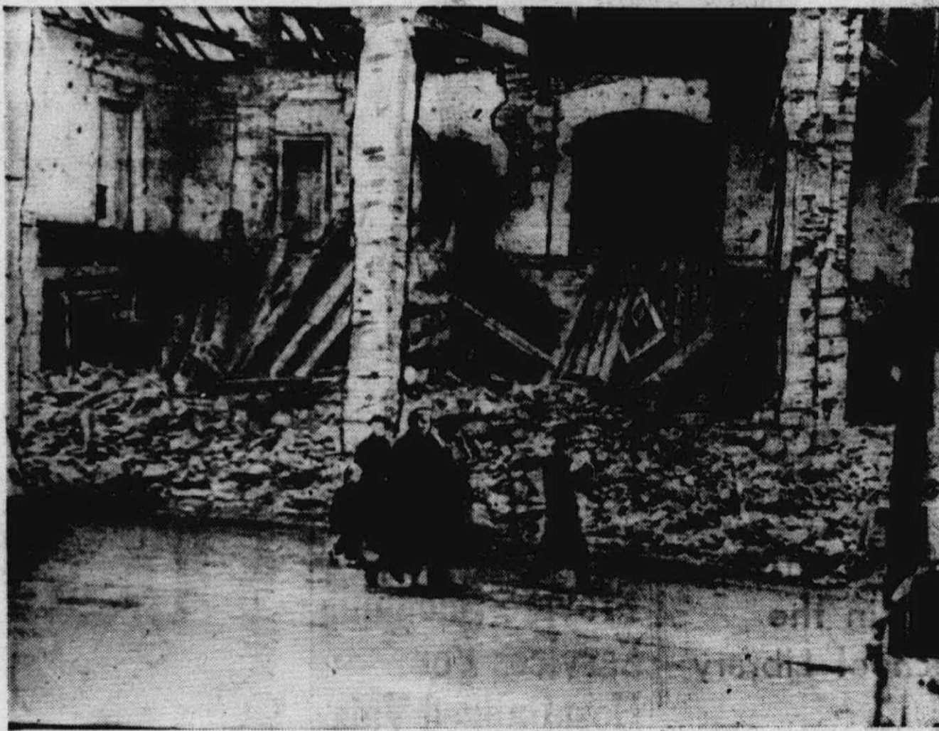
RED RUIN . . . Hungarians face task of rebuilding revolt-torn Budapest to provide winter shelter for hundreds and to enable industry to resume operation.
