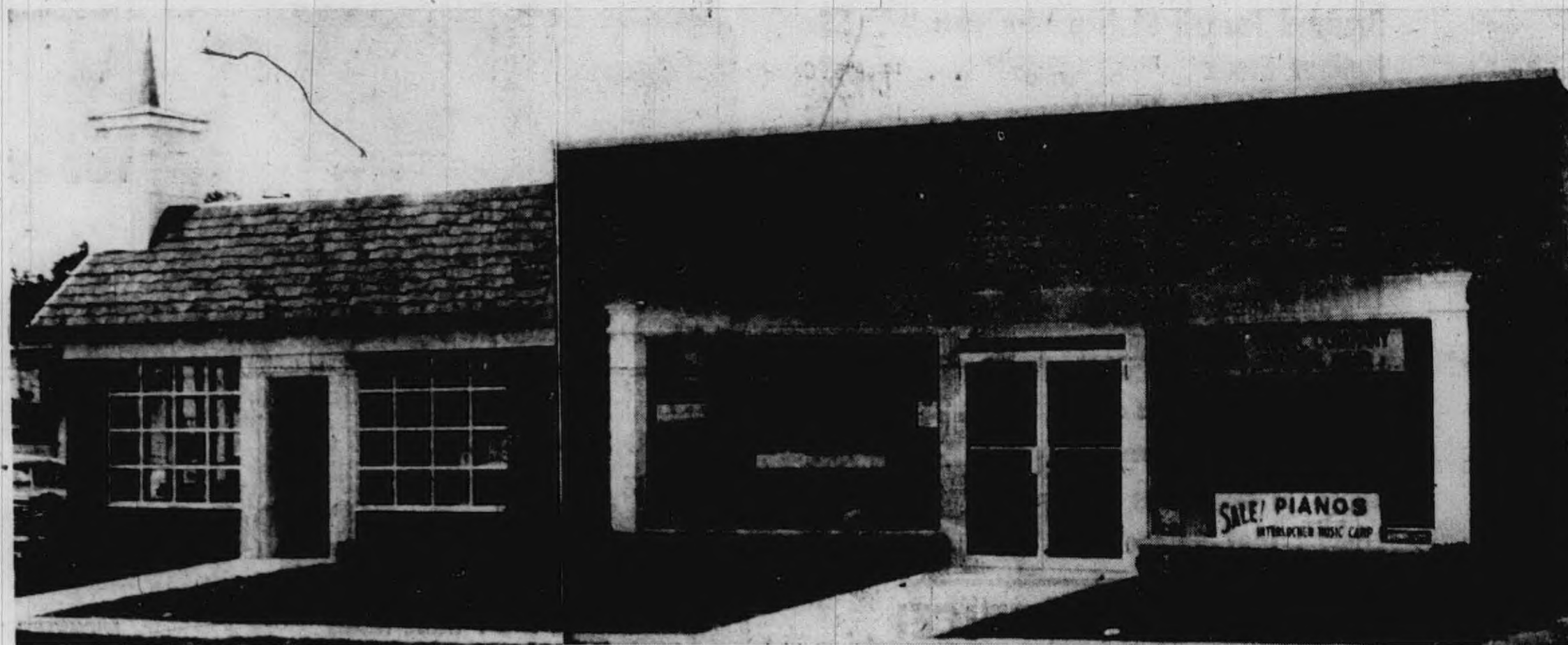
This modern, spacious new commercial building at 504-518 S. Main St. in Plymouth, exemplifies the trend to colonial design in the downtown area. We, as contractors, are proud to have had a part in erecting this building. The C. L. Finlan Insurance office will be ready for occupancy early in October.
