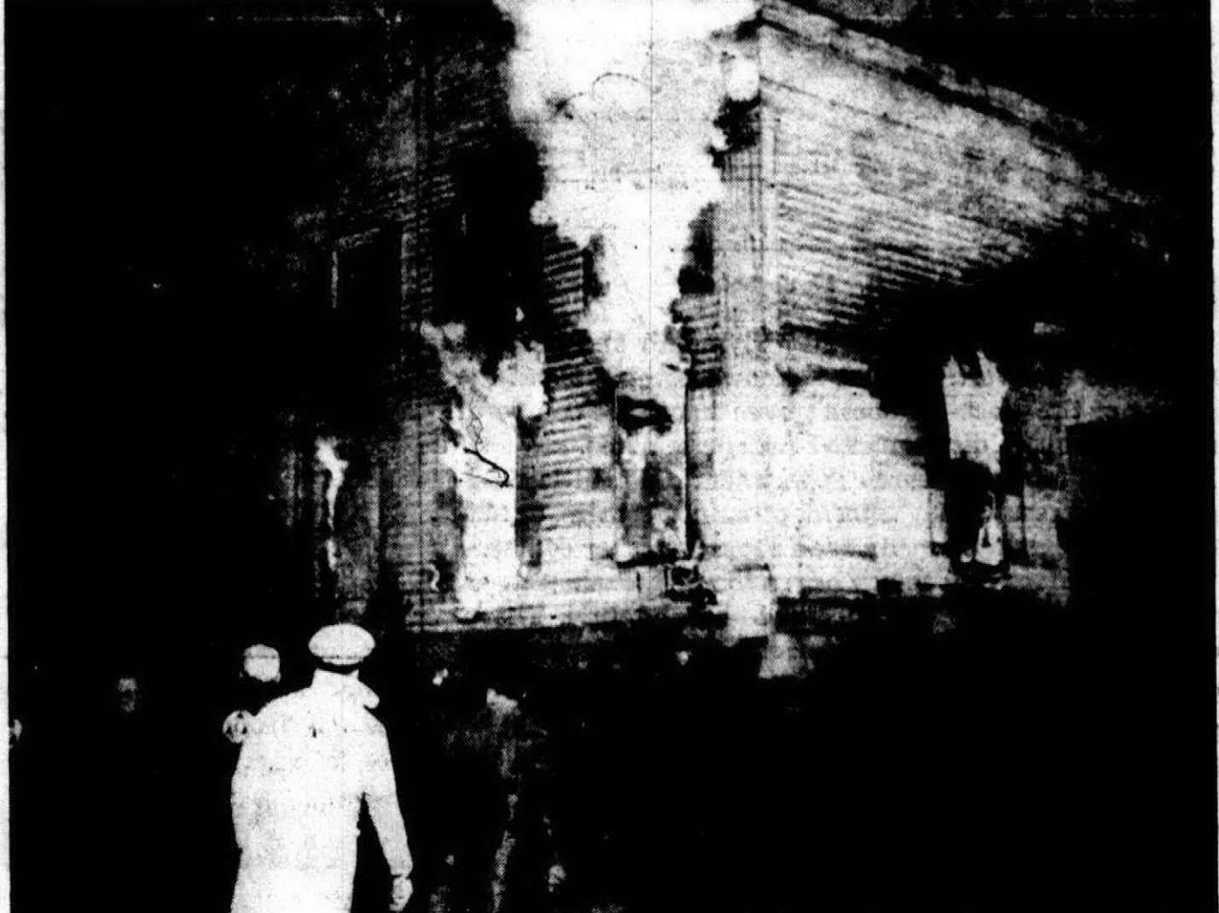
FIREMEN FROM FIVE departments battled this blaze recently near Novi and Novy. It was being burned to make way for the Lincoln plant. Practicing their fire-fighting skills were firemen from Plymouth city, Lyon township, Novi, Northville and Salem township. Chief Robert McAllister (in white coat) and several local firemen are seen in foreground.
