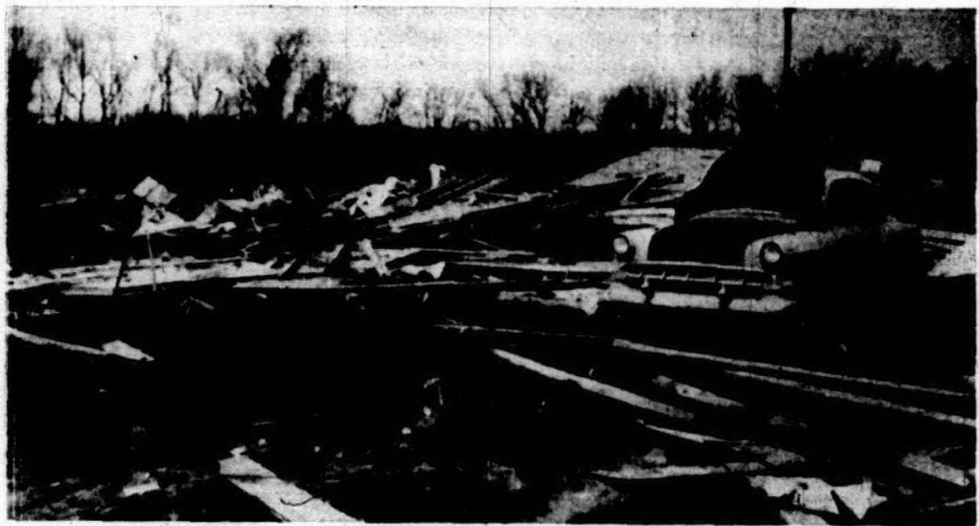
MOST VIOLENT damage caused by the storm in this area occurred in South Lyon. The above home of Mr. and Mrs. Harlan Bryant was leveled Saturday as was a newly built home next door which the Bryants planned to move into Sunday. The Bryants and their eight-week-old son were in the home when the wind struck but escaped with minor cuts. Bryant is employed at Evans Products in Plymouth.
