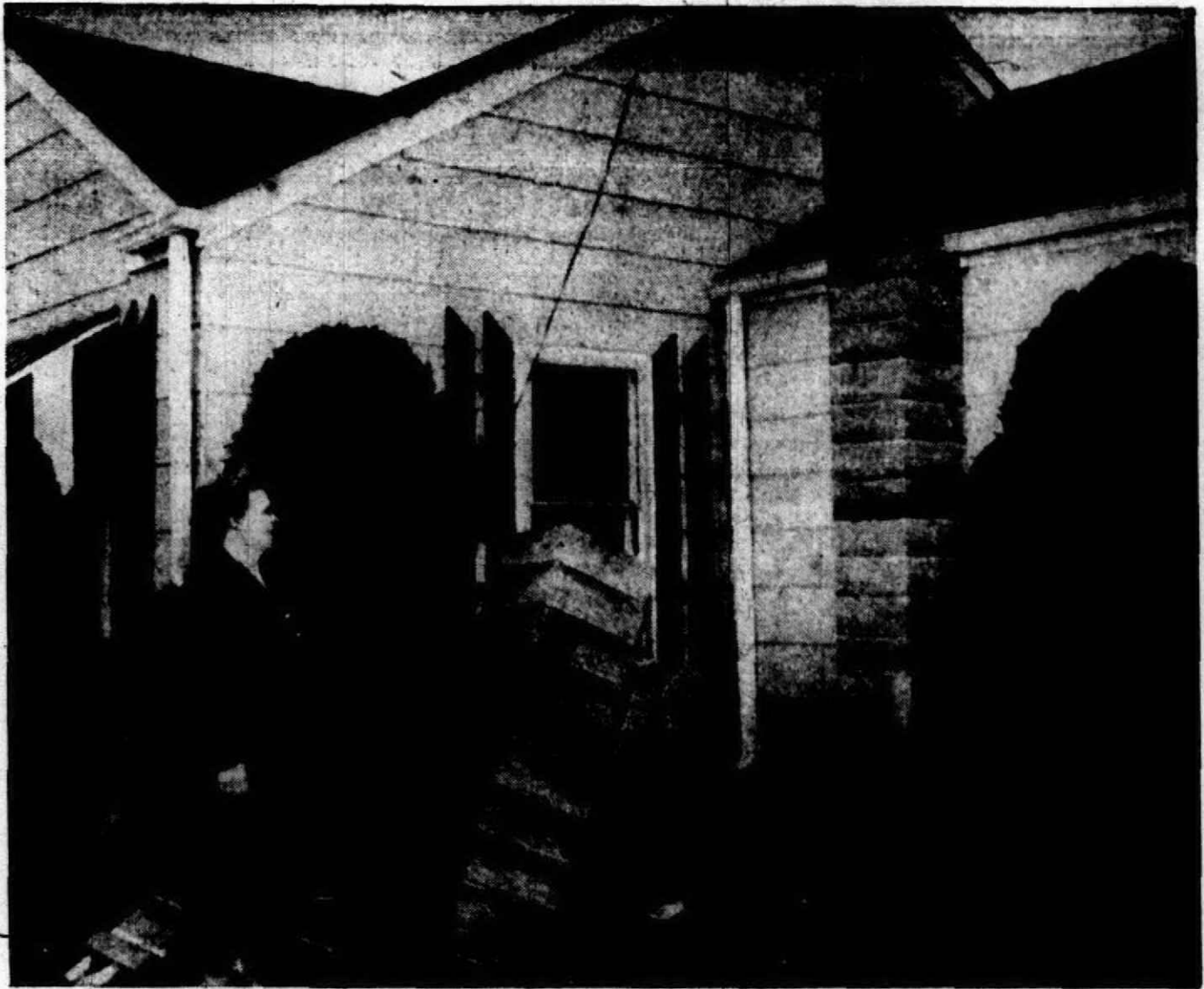
MRS. ALBERT Minehart of 8911 Brookline examines top portion of the chimney which was blown from the house shortly after 6:00 p.m. Saturday. The Mineharts reported that the strong winds shook the house and crashed the chimney into the ground as they watched from a nearby window.
