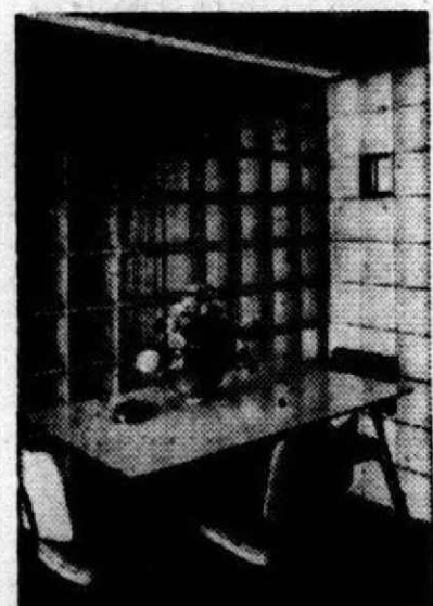
A bright and cheery dining area is set off with an interior partition of glass block. The exterior wall which gives light and privacy both is shown with glass block ventilation.
