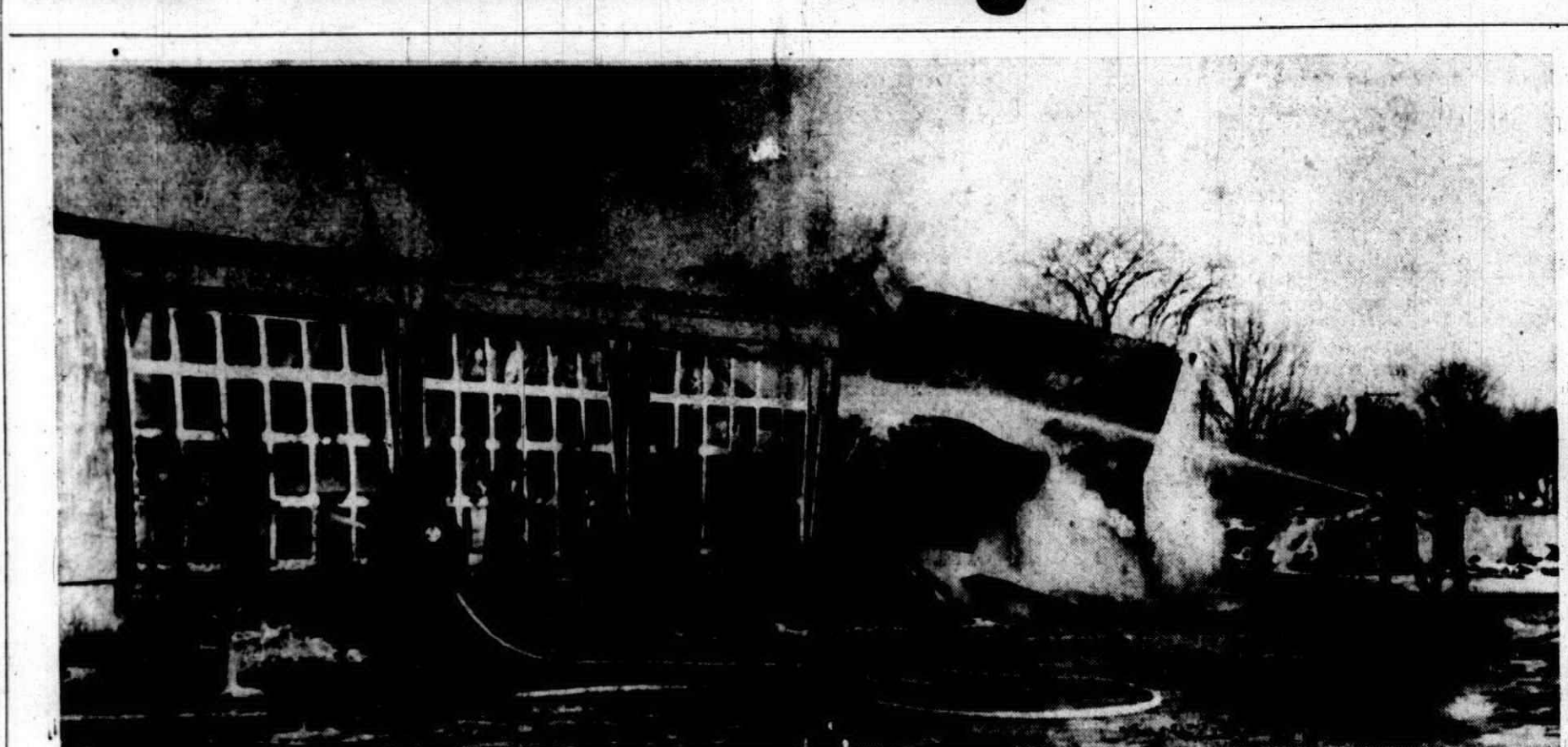
WALLS OF the Warm Air Heating Supply company warehouse crumble and collapse as firemen battled the blaze yesterday morning which destroyed the large store house at 9800 Ann Arbor road. Within the building and also mostly consumed by the flames were stored heating
