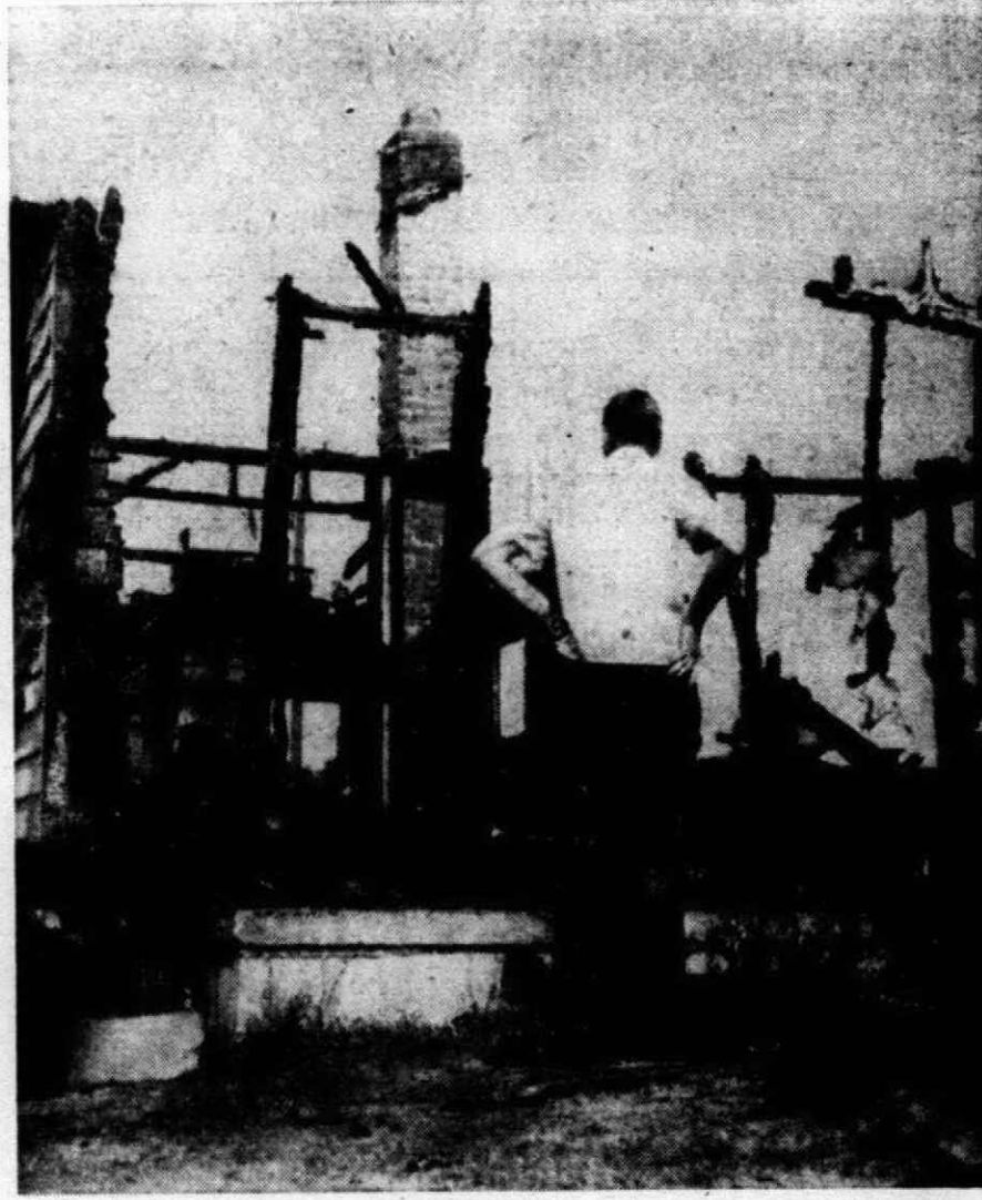
THREE CHILDREN died in this fire last July when the home of Calvert Montgomery on Maxwell burned to the ground. The tragedy was the worst in the area during 1955.
