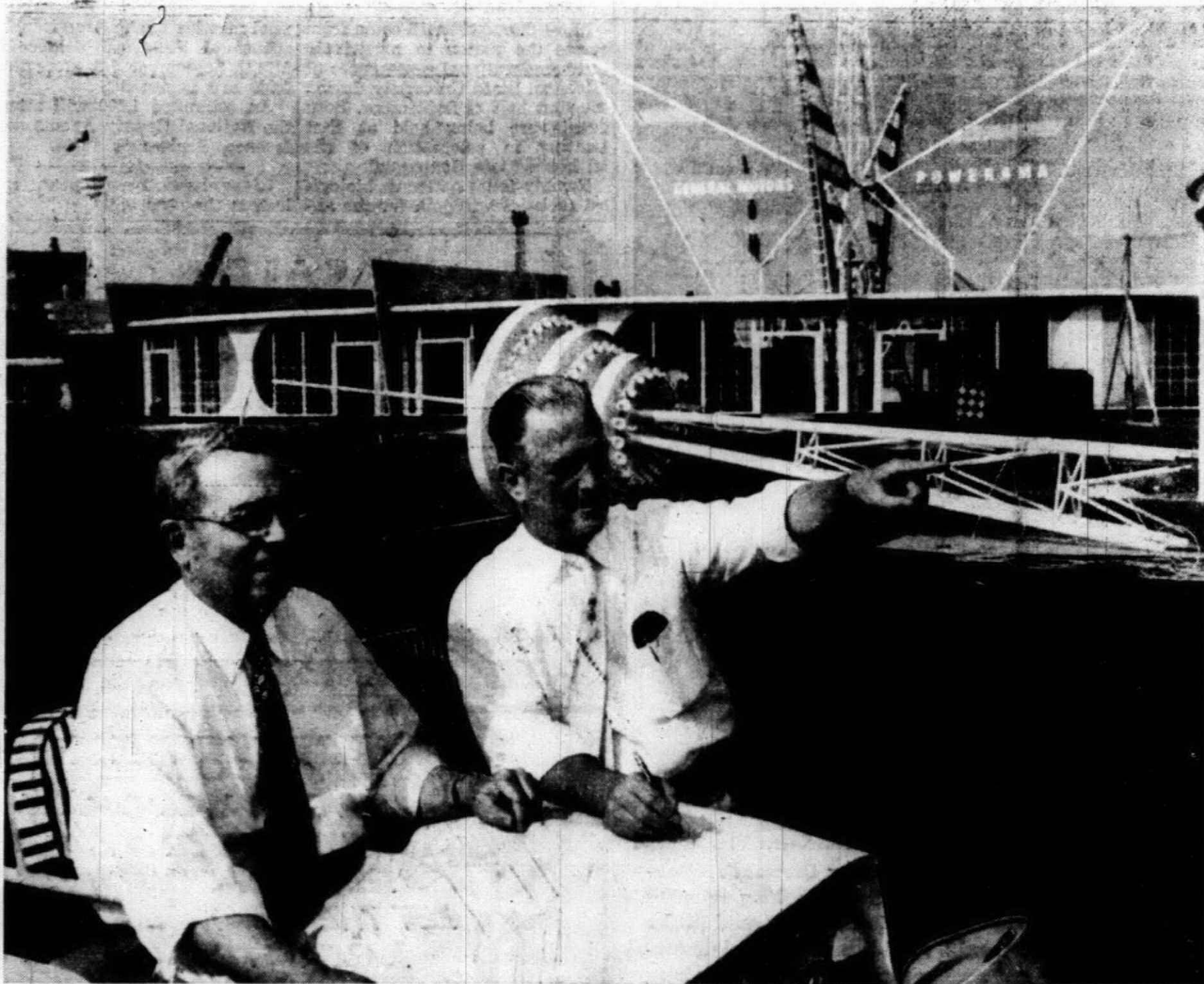
PLANNING POWERAMA CONSTRUCTION are Spencer D. Hopkins (left), director of General Motors Sales Section, and Plymouthite T. H. Roberts, Powerama manager. The two men have the responsibility for the entire building and operation of the giant "world's fair
