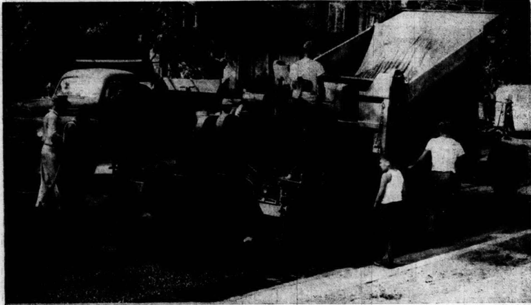
THE ACTUAL PAVING of Plymouth's newly widened Main street got underway Monday with company officials reporting that the resurfacing should be completed this week. Pictured above the hot-mix asphalt is being fed into the paving machine, which in turn
