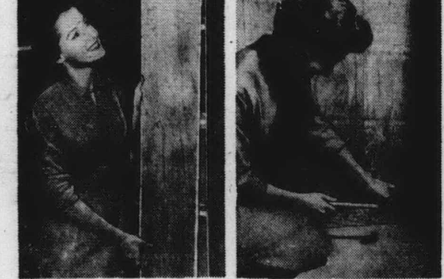
Lock panels firmly to row of clips. Finish your paneling with moldings and trim of matching oak.
