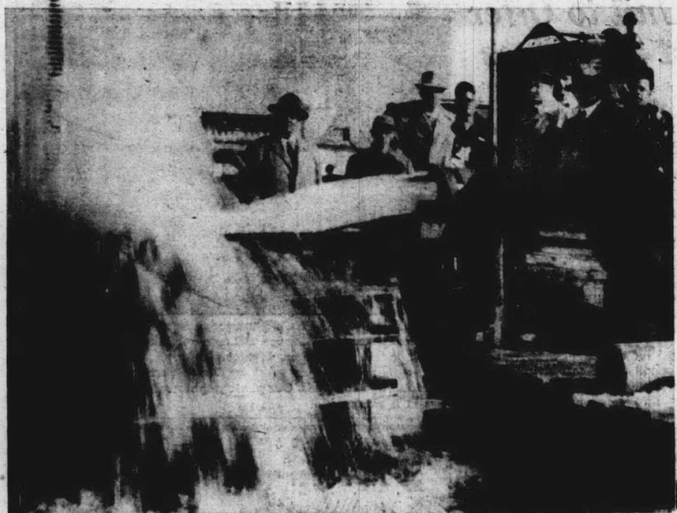
A RESERVE water supply capable of taking care of Plymouth's needs in the hottest of weather was forecast last week as drillers tested a new well on Six Mile road near Beck. Shown above is the well being pumped out at the rate of 5,000,000 gallons a day as city officials, consulting engineers and drillers watch. Present pumping facilities and pipe sizes will allow the well a usefulness of only 1,000,000 gallons a day. It will be several months before the new well is actually hooked into the present system. At side is a view of the "screen" being lowered into the 18 inch hole, one of the largest screens used in water well drilling. The hole is about 110 feet deep and is located a short distance from present well field.
