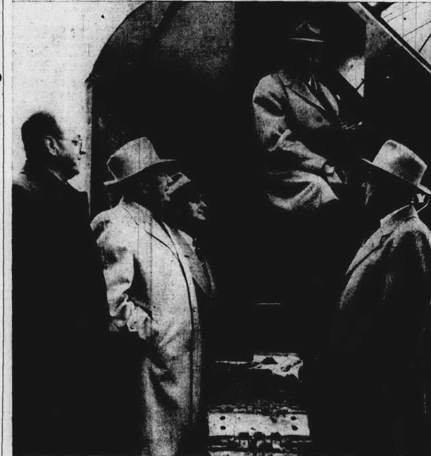
A POWER SHOVEL replaced the usual spade at ground-breaking ceremonies last Wednesday at the site of the new National Bank of Detroit office, Ann Arbor road and Harvey street. Shown are Mayor Russell M. Daane, member of the bank's Plymouth-Livonia advisory committee, in the cab of the shovel, who is chatting with (left to right) Floyd A. Kehrl and Harry O. Mohrmann, vice-presidents; Jack E. Taylor and Harry Larsen, assistant vice-presidents. The modern bank will have 2,000 feet of floor space, air conditioning and two drive-in windows.
