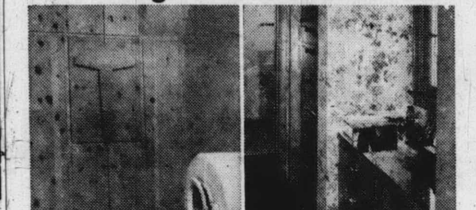
This built-in for a laundry area has many possible uses elsewhere. Door swings down as a table.
