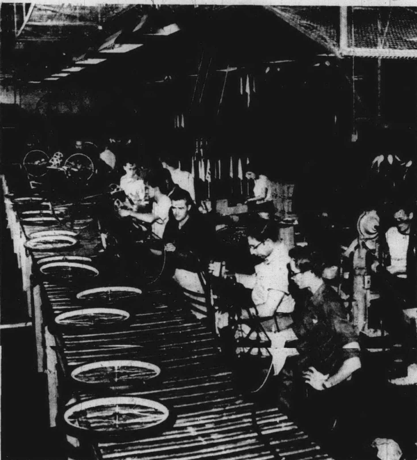
OVERHEAD CONVEYORS speed up production at Evans products. Here velocipede semi-assemblies approach the final assembly line. Velocipedes were designed by Harley Earl, design genius of General Motors.
