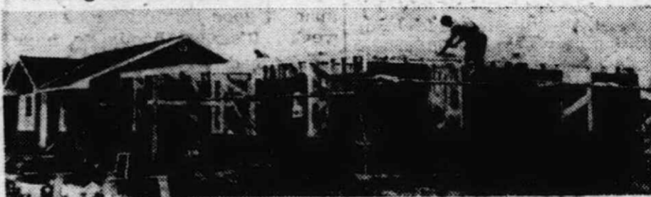
When insulating siding and gypsum board sheathing are used together as they are in this housing development, the home owner gets several "bonus" values. Not only is the cost lower, but he gets the benefit of additional protection from the fire resistant gypsum board, and insulation from the siding.
