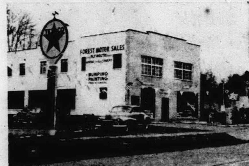
906 S. Main — Our PLYMOUTH Showroom GAS STATION and BODY SHOP
