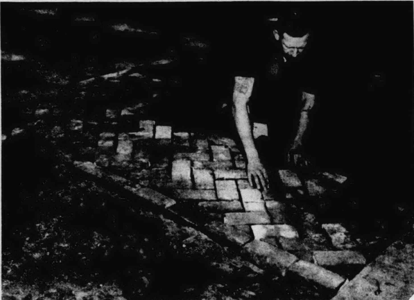
A NOVEL DO-IT-YOURSELF PROJECT is shown being completed by Grayson Jones of 1424 W. Ann Arbor Trail. The first in a series of lawn decorating schemes being planned by Jones, this used brick walk is being laid between the road and the sidewalk. A project of this sort is both decorative and inexpensive for the homeowner to utilize in adding to the charm of landscaping.
