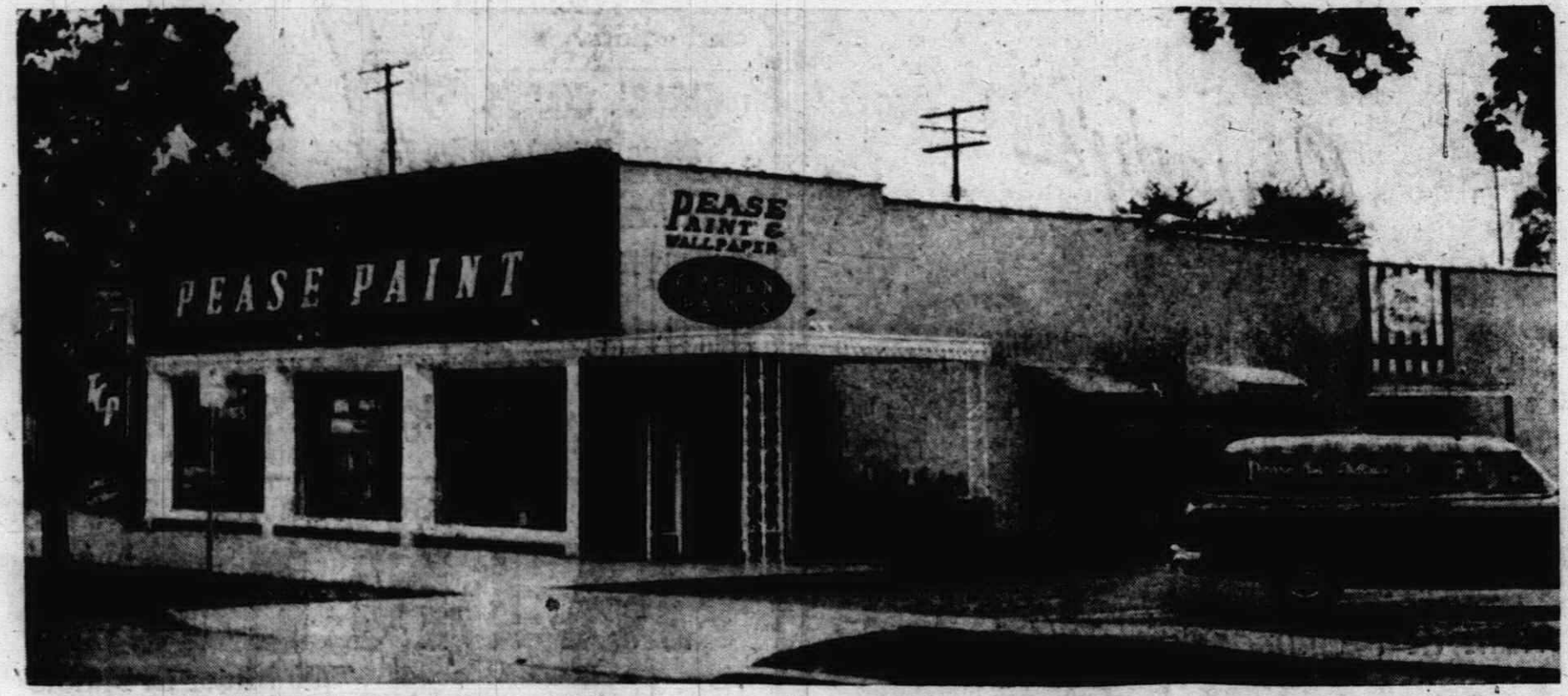
THE NEW HOME of Pease Paint & Wallpaper company at 570 South Main street was designed in the modern colonial style to conform with Plymouth's theme. A 10-day Grand Opening celebration starts today.
