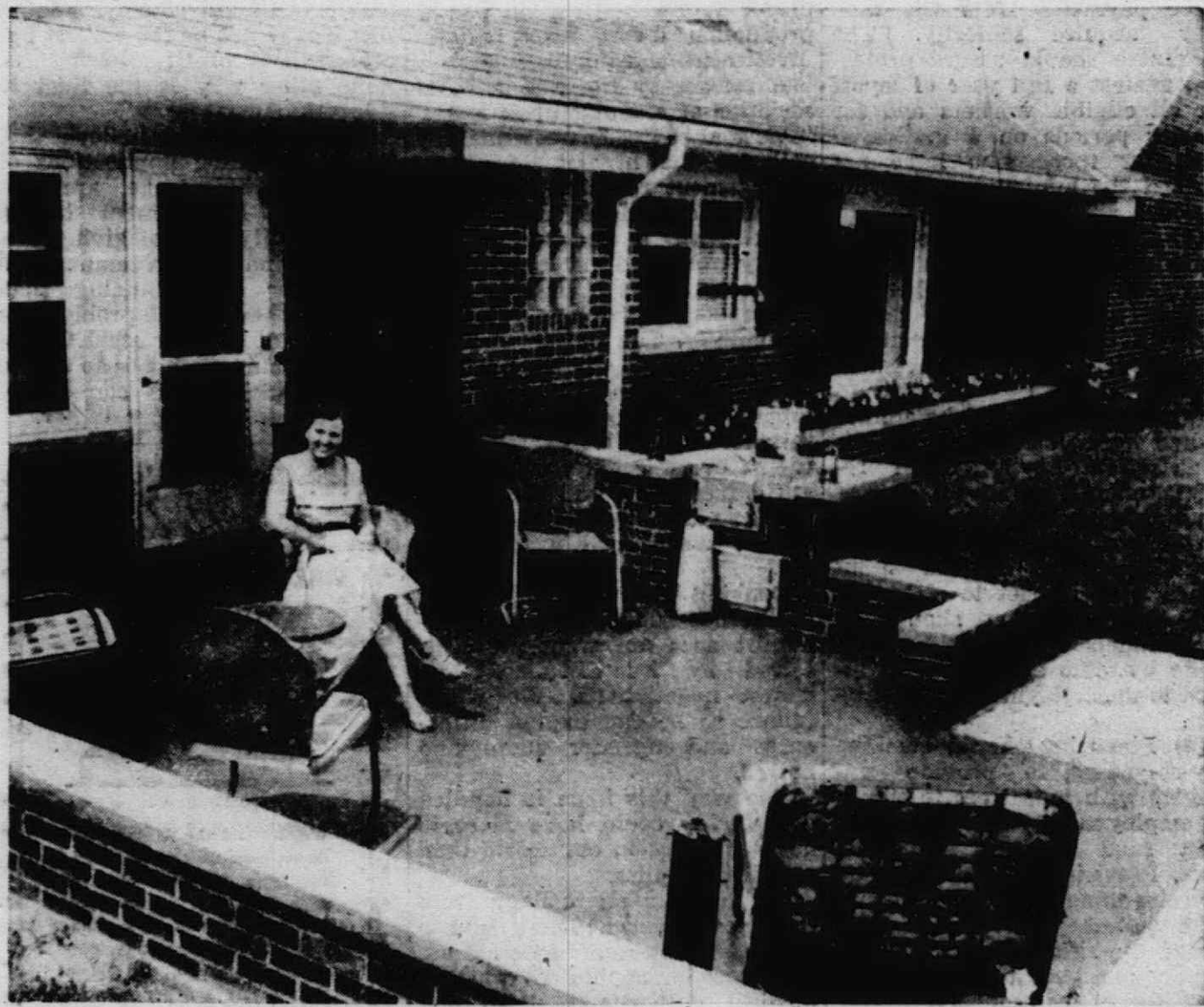
A real do-it-yourself project for the Jack Gage family of 42501 Clemons road is this terrace at the rear of their home. Mr. Gage and their son, Jim, hauled the cement and put up the brick wall, all from their own design. They even built forms and poured the cement for the ledges. Green cement paint is used on the floor, and the terrace features a built-in fireplace.
