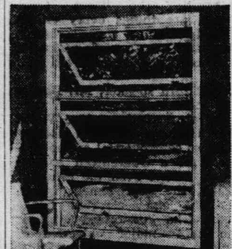
Awning-style window opens outward, keeps rain from entering.
