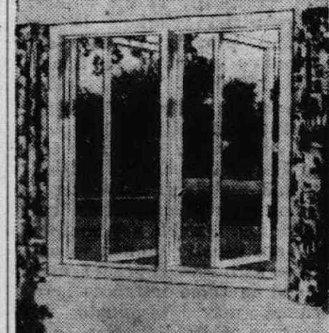
The same sash in a vertical position becomes a casement window.
