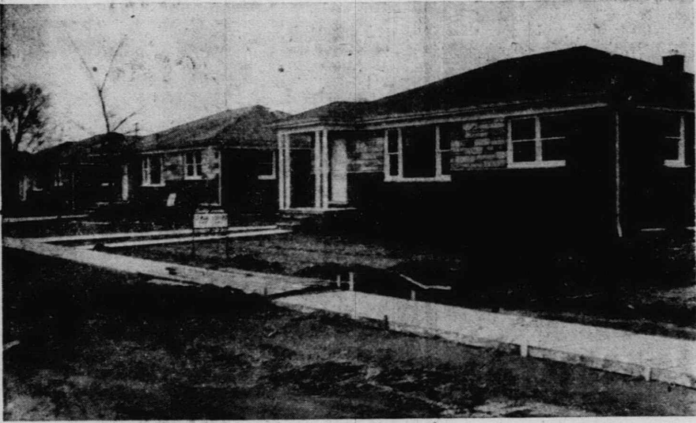
ONE OF THE MAJOR contributors to the "new look" on Simpson street is Contractor Stewart Oldford. Three of his homes are shown above and others may be found in the Smith school area making it one of the nicest, new residential sections in Plymouth. Featuring three-bedrooms, Oldford's homes offer modern, ranch-style design and latest features for maximum home comfort.
