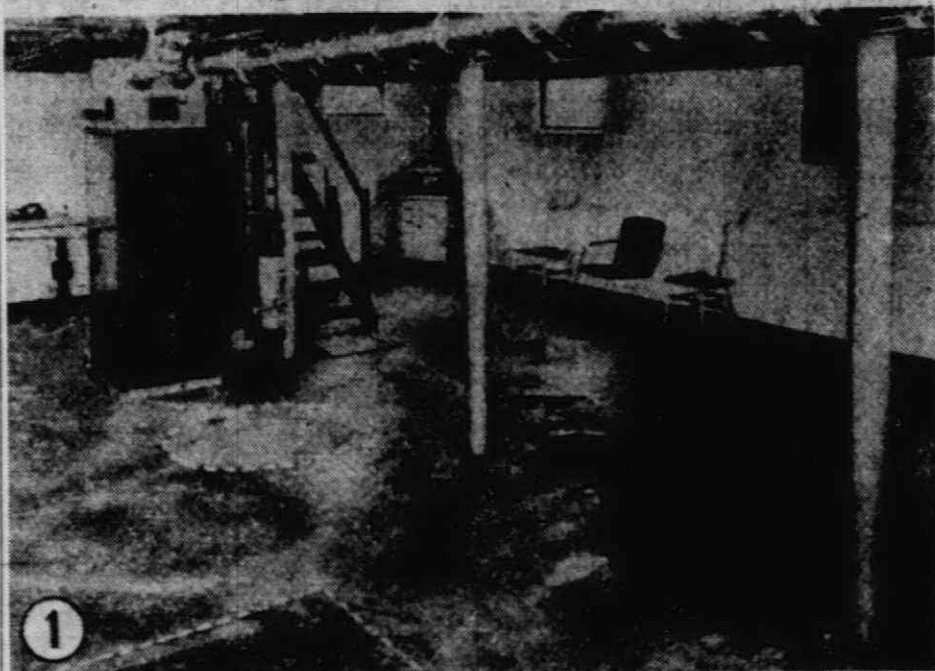
Space formerly taken up by old furnace and coal bin is outlined in dotted lines. New furnace fits snugly against chimney and modern heat-ducts are well above head level.
