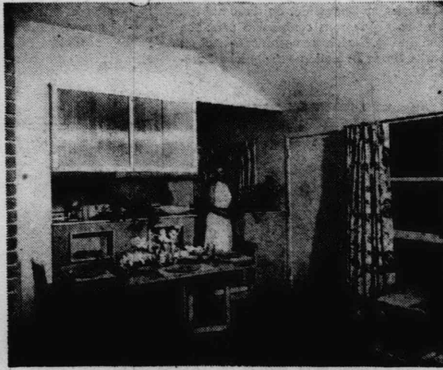
A pass-through between the kitchen and the dining area saves many dozens of steps a day in serving meals. The pass-through illustrated here has a convenient hanging cupboard above the usual counter. All the dishes and silver needed for a meal can be laid on the counter from the kitchen side and then can be easily reached from the dining room side later. A hanging cupboard of this type can have doors on both sides.
